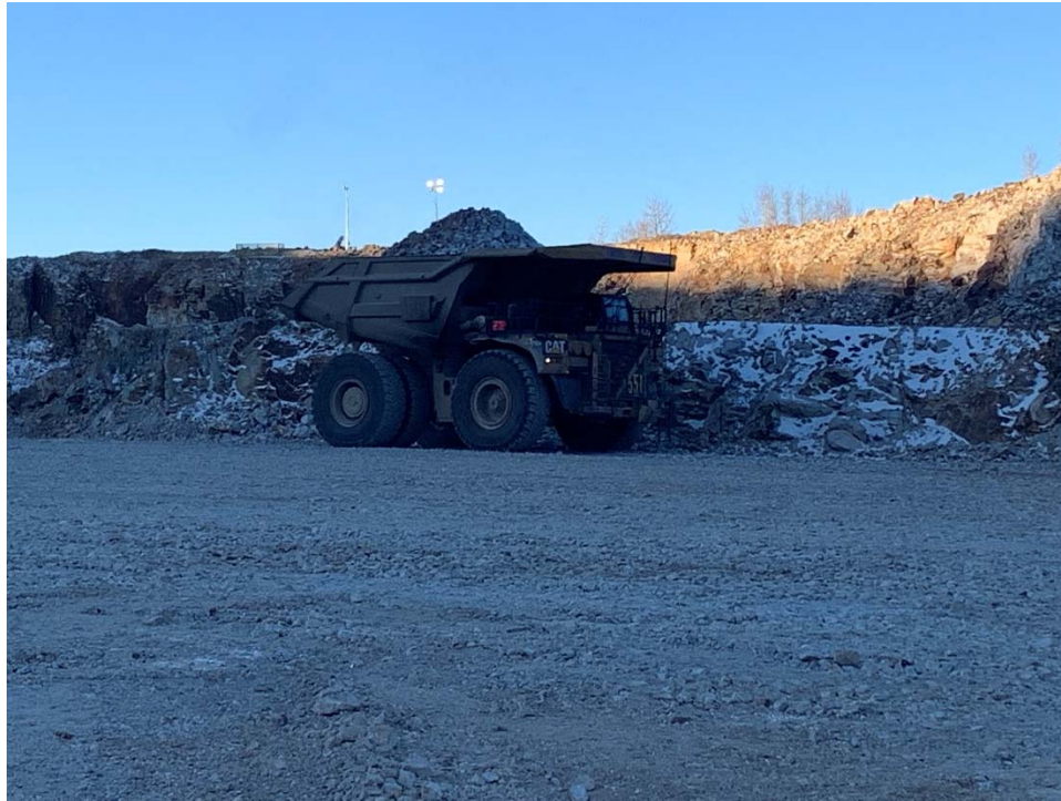
December 17, 2021 – High Compaction Backfill wheel rolling (TW)
