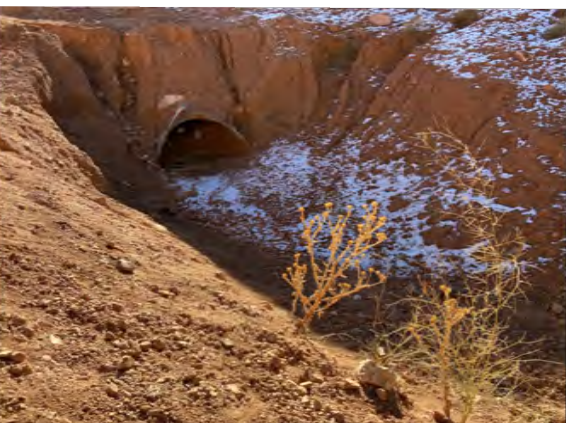
3. UPSTREAM END OF CULVERT WITH PIPE
