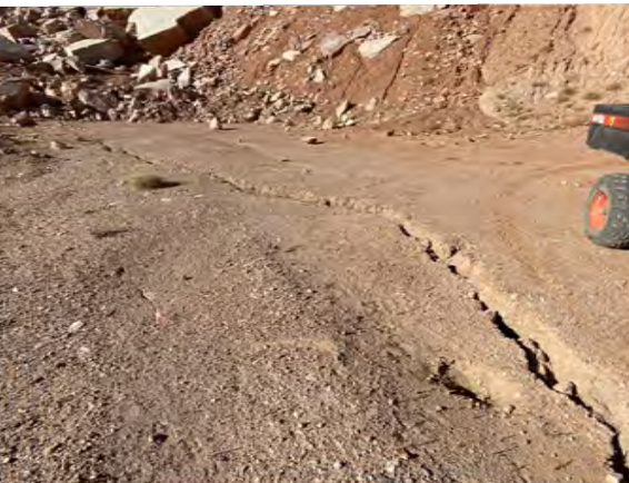
2. CRACKING NEAR PRODUCTION FLOOR
