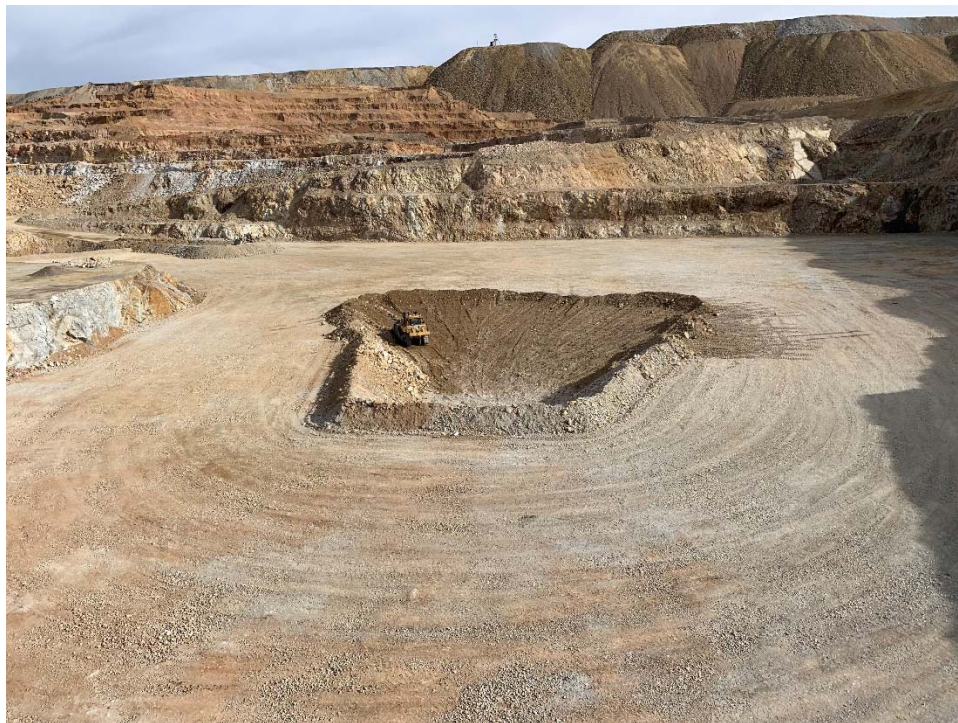
December 1, 2021 – High Compaction Backfill cut contouring (TW)
