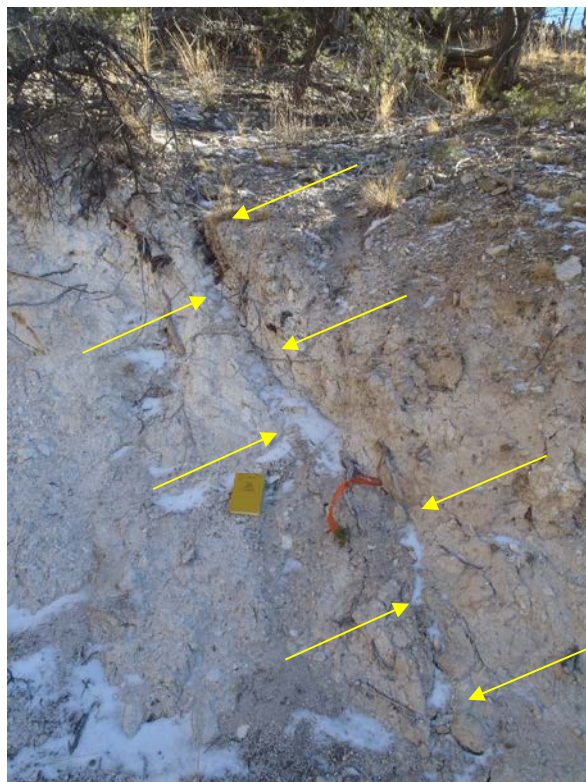
Photo 4. Tension crack viewed in access road cut, ~100 feet NE of dozer (looking east).
