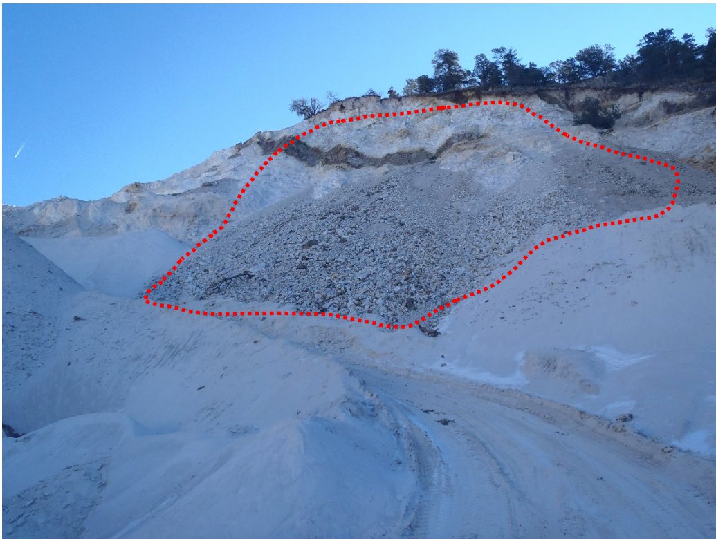
Photo 2. Second 2021 failure (north facing slope, looking east from pit floor)
