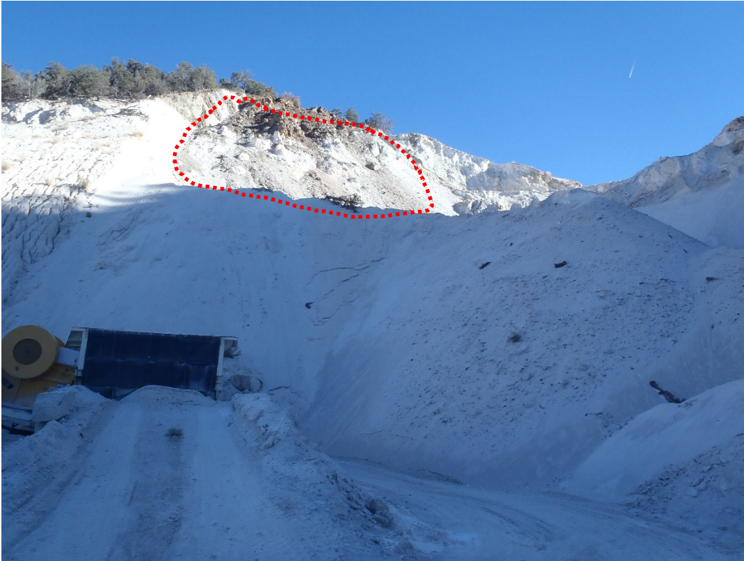
Photo 1. First 2021 failure (south facing slope, looking NE from pit floor).
