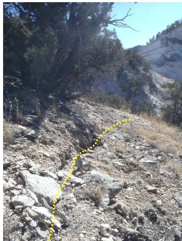
Photo 6. Tension crack viewed SE of access road/dozer trail (looking SE, north facing highwall beyond).
