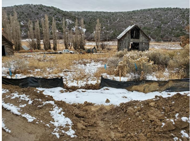
Photo 8: Sediment trap at bottom of LCC access road As road opens up to Old Barn work area
