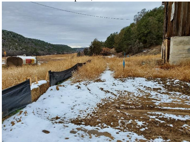
Photo 6: Old Barn area, LPCR 120 on L side of photo Silt fence and hay bale sediment control in good repair. Looking southwest
