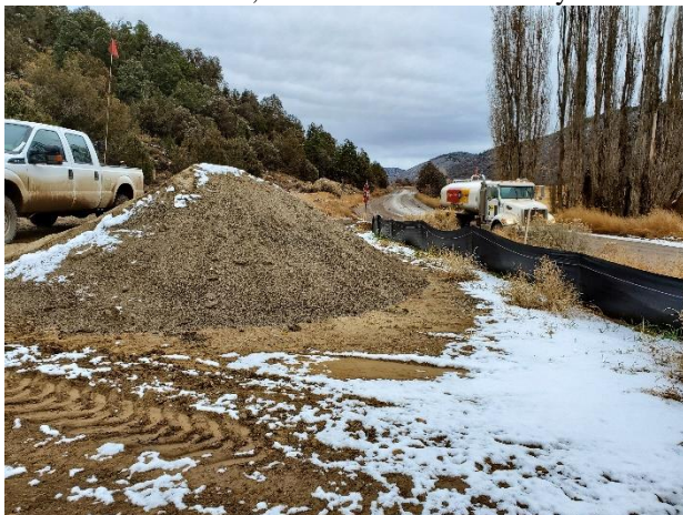
Photo 5: material stored upslope of sediment fence at Old Barn area. Looking northeast
