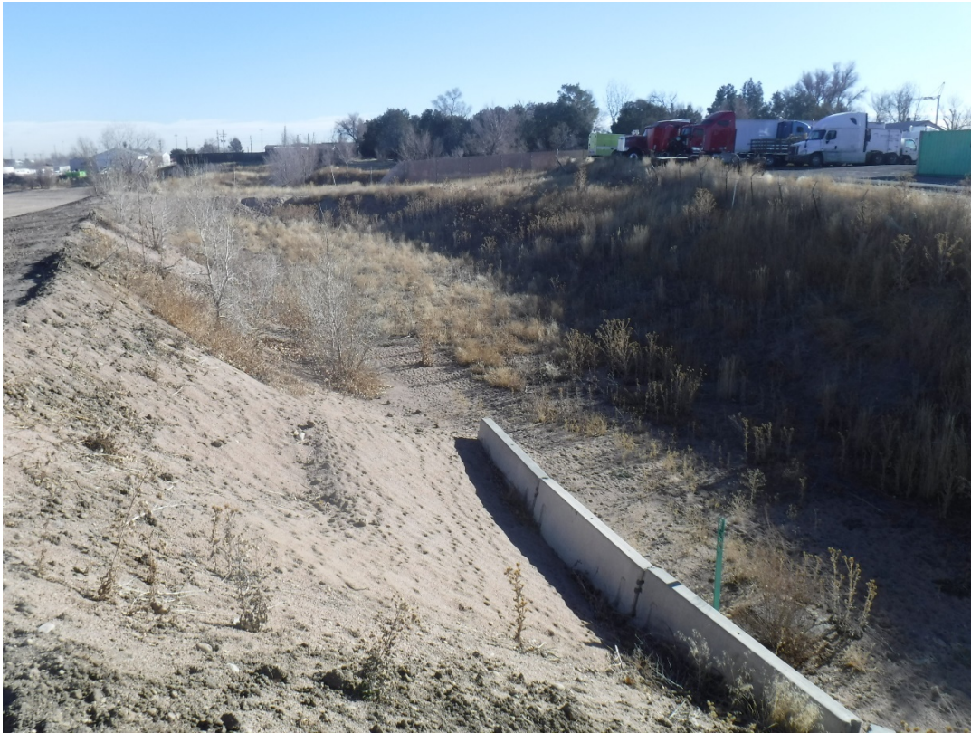
Photo 7: South side of the southern berm not graded to 3:1
