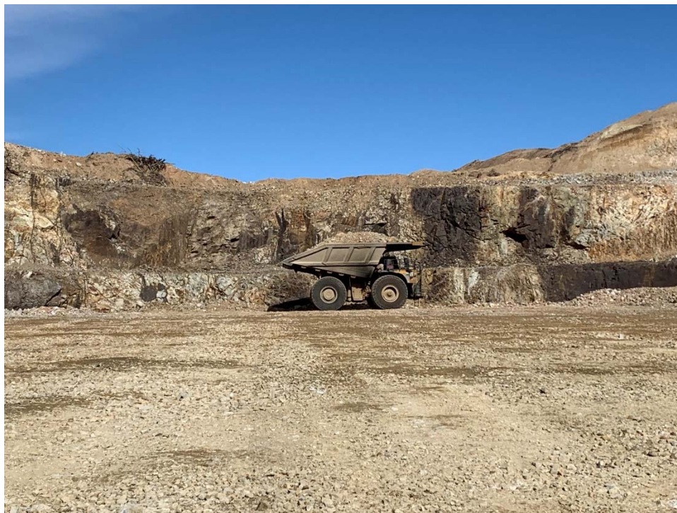
November 11, 2021 – High Compaction Backfill wheel rolling (TW)
