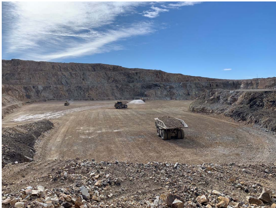
November 11, 2021 – High Compaction Backfill wheel rolling (TW)
