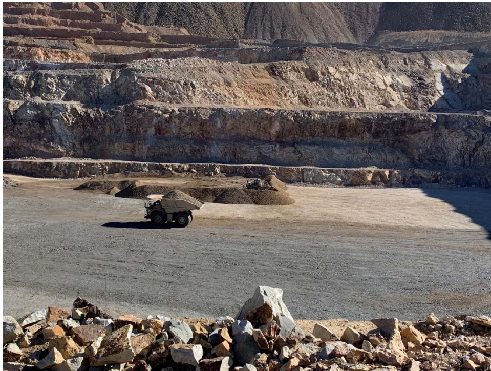
November 7, 2021 – High Compaction Backfill placement and wheel rolling (TW)
