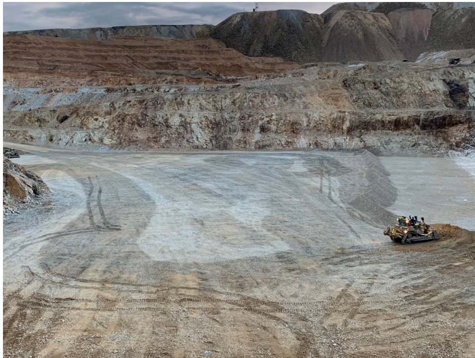
November 24, 2021 – High compaction backfill placement (TW)
