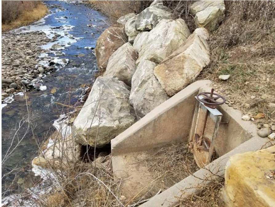
Figure 3. Rip-rap placed on river bank upstream of the outlet of Pond 004.
