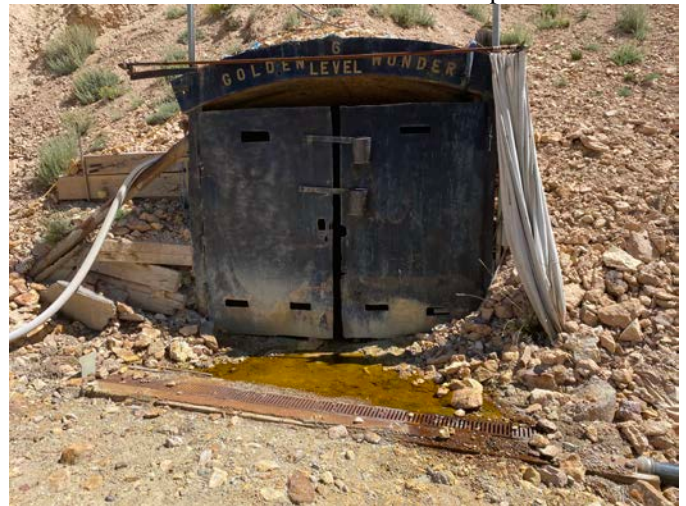
Level 6 Portal with Subsidence/Collapse above
