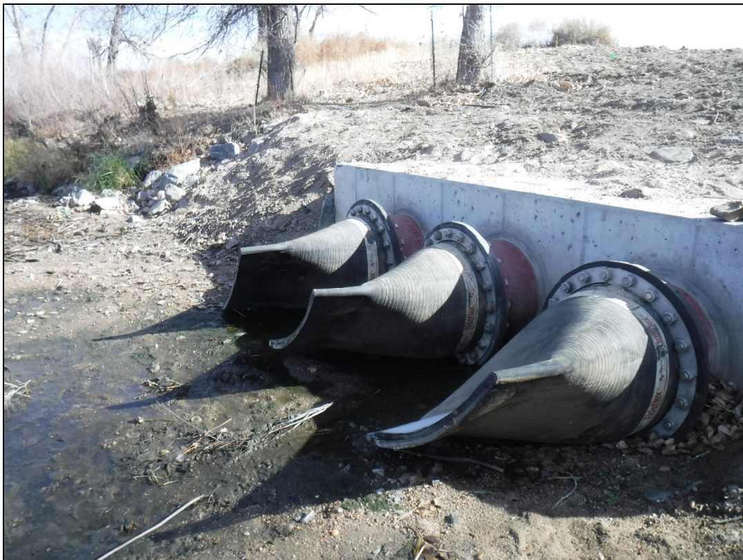
Photo 10: Culvert outfall points to Platte River
