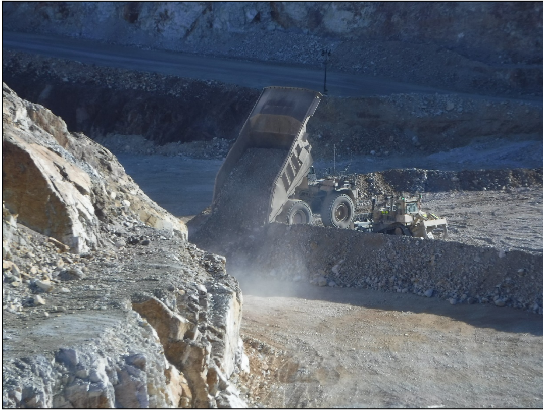
Photo 5: End dumping of material
