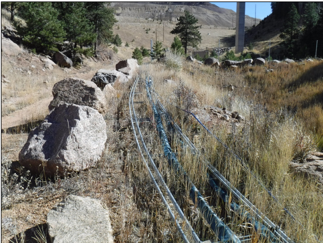
Photo 22: CRMW-3 series wells discharge tubing and electrical conduits
