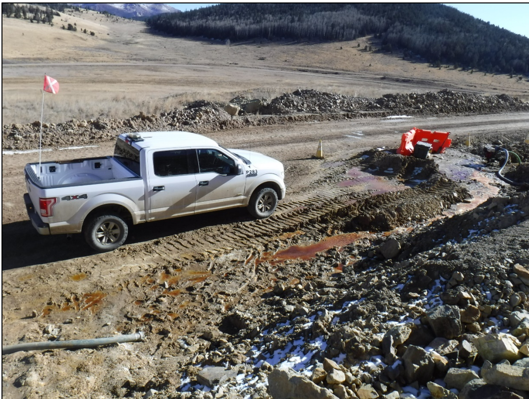
Photo 8: Pumping set up to remove seep water from the seep 2 area
