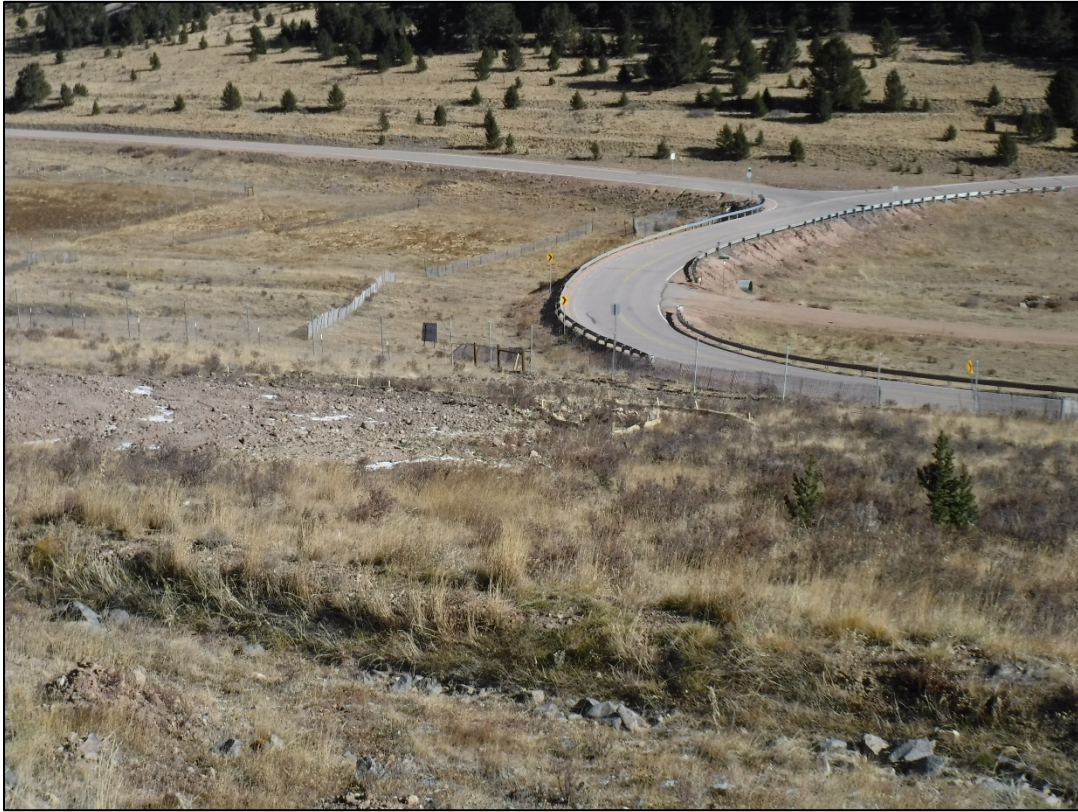
Photo 11: Reclaimed drill pad area with stormwater controls in place downgradient of pad and sediment has been removed from wildlife fence
