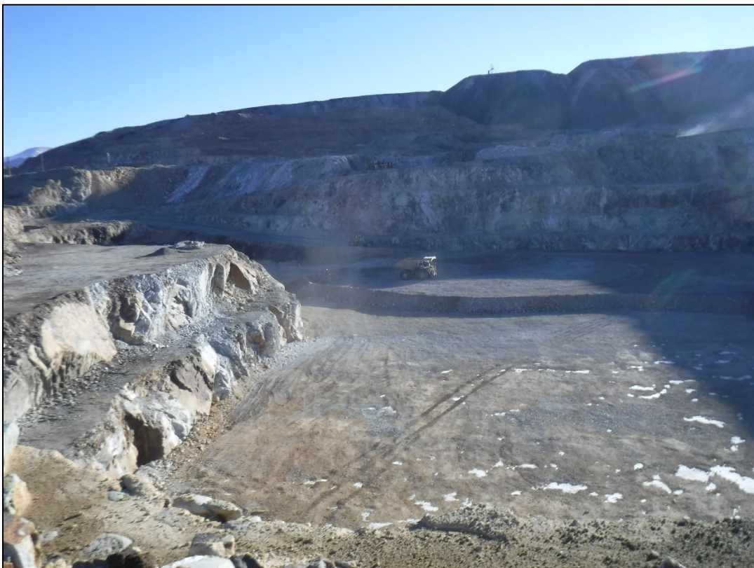
Photo 2: Schist Island high compaction area first 5 foot lift
