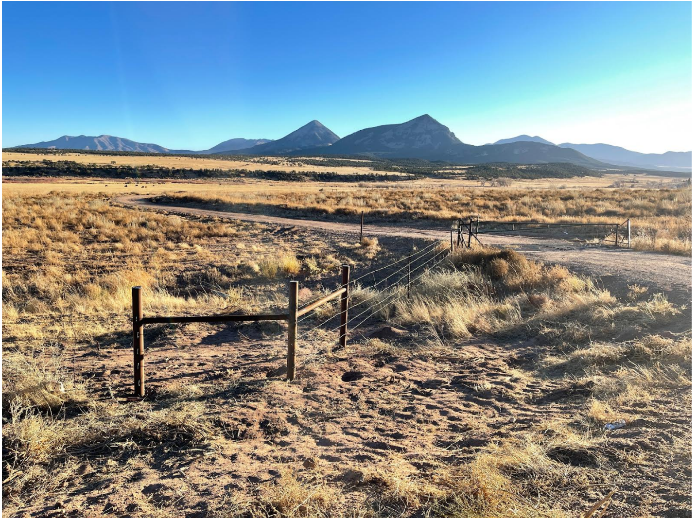
Looking south west at new road under dam and reservoir east gate
