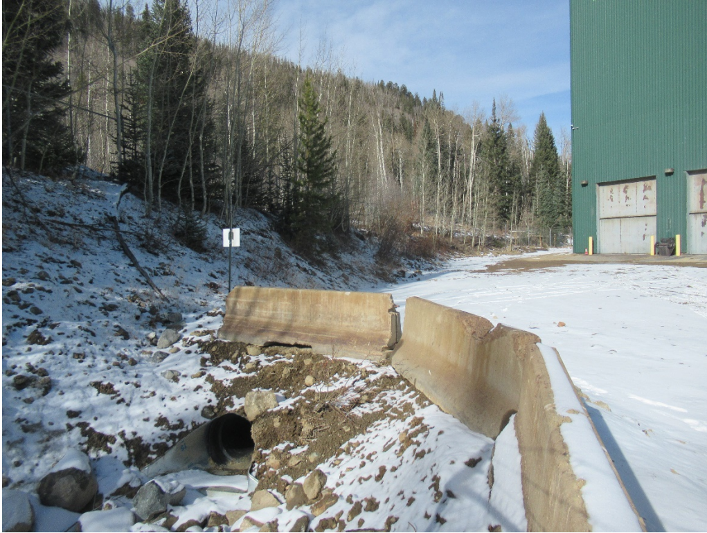
View of the piped section of the stormwater ditch located southwest of the PC2/PC3 transfer station
