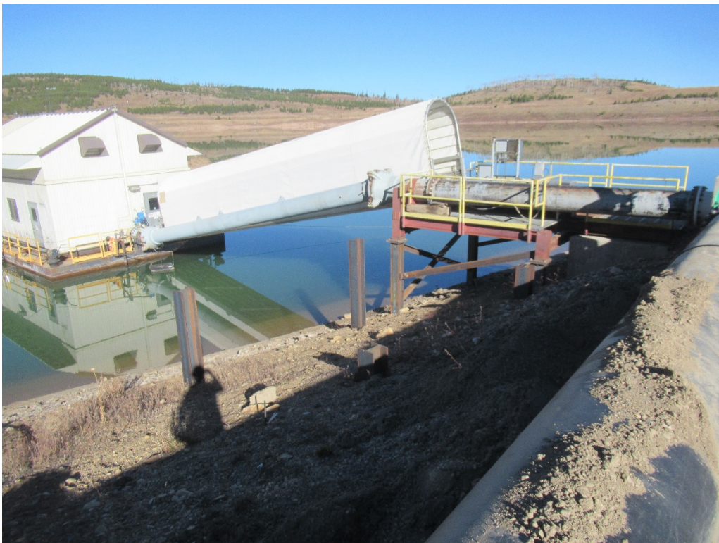
View of the two new foundations for the barge
