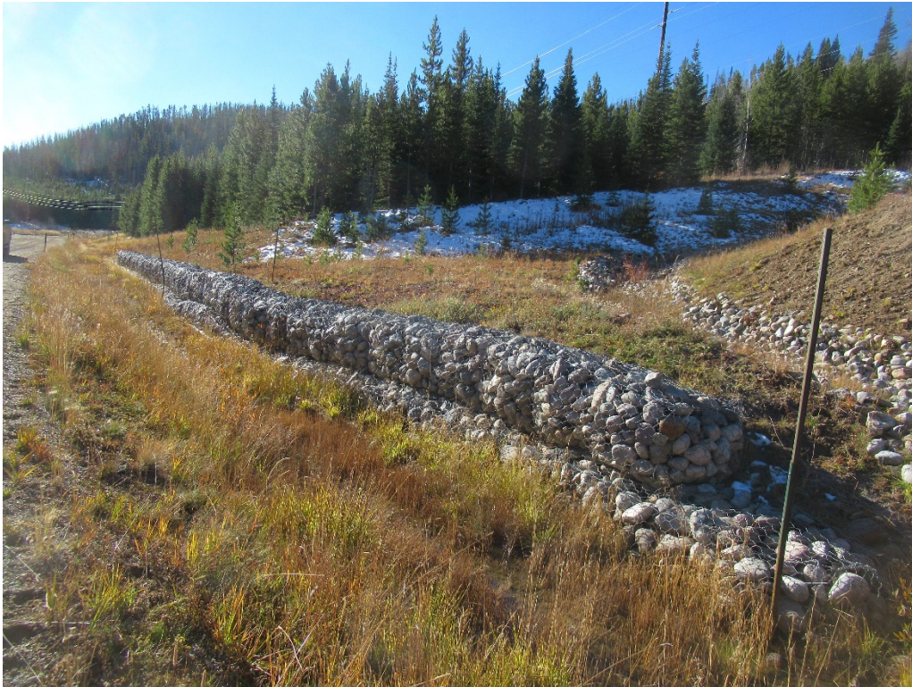
View of gabion structures along the ultimate canal
