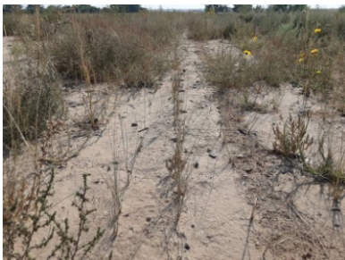
Haul Road: Desirable vegetation in isolated locations of haul road (photo 8) Consider selective ripping and reseeding in this area
