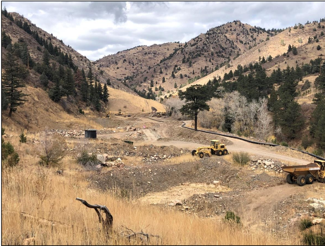
Photo 1. View looking northwest (from top of mesa with water treatment plant) across northwestern valley excavation project area. Excavated soils are currently being disposed of inside Black Forest Mine, per AM-5.
