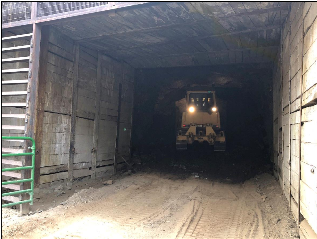
Photo 8. View looking inside Black Forest Mine, in which, excavated soils are being placed, per AM-5. At time of inspection, toe of backfilled material was approx. 50 feet from mine entrance gate.
