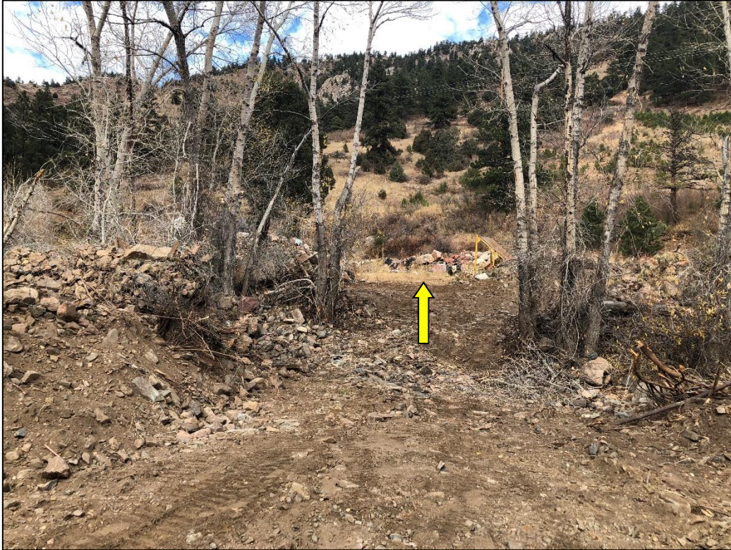
Photo 11. View looking east at new access (indicated) to storage area located north of creek, as existing bridge access is restricted by adjacent excavation activities.
