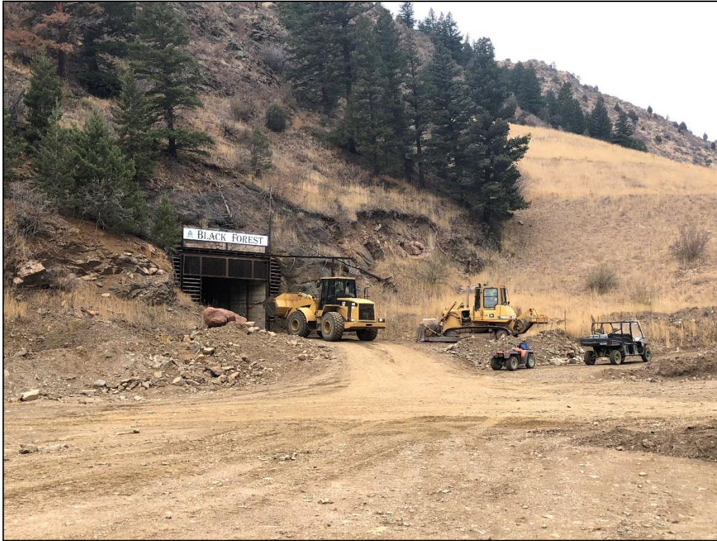
Photo 7. View looking northwest at main entrance to Black Forest Mine, in which, excavated soils are being placed, per AM-5.
