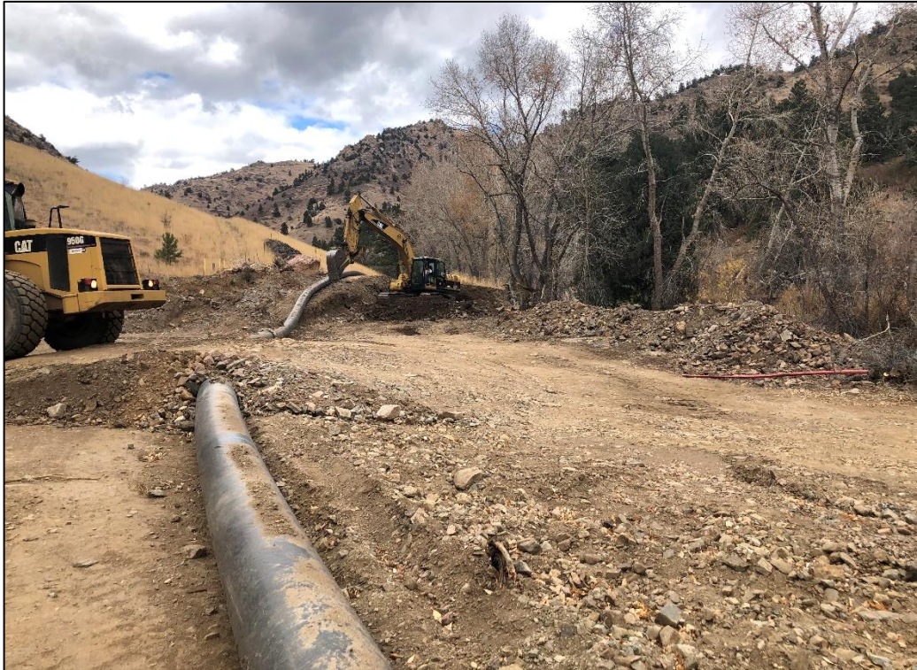
Photo 5. View looking north at current excavation activities (in northwestern project area) adjacent to southeastern toe of SWRP (slope visible left of excavator). Note bypass pipeline (in foreground) temporarily relocated.
