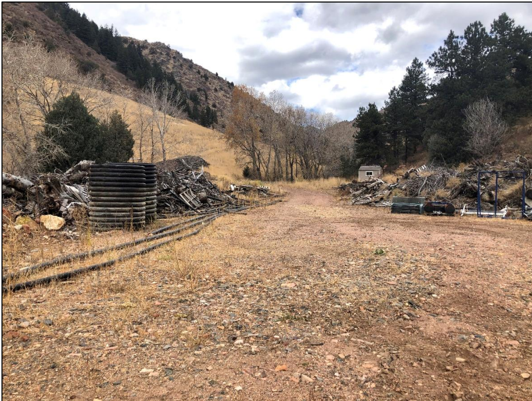
Photo 12. View looking northwest across storage area located north of creek showing woody debris, rocks, and various pieces of equipment and empty storage containers stored in this area. All equipment will be removed from this area. Woody debris will be chipped for mulch, and rocks will be used for reclamation backfill.
