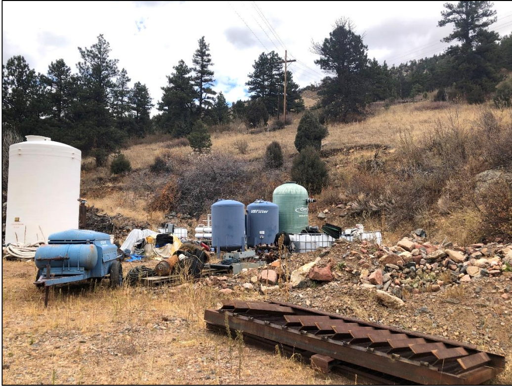
Photo 13. View looking east at storage area located north of creek showing woody debris, rocks, and various pieces of equipment and empty storage containers stored in this area. Adjacent undisturbed hillside (in background) may be used as a topsoil borrow area.
