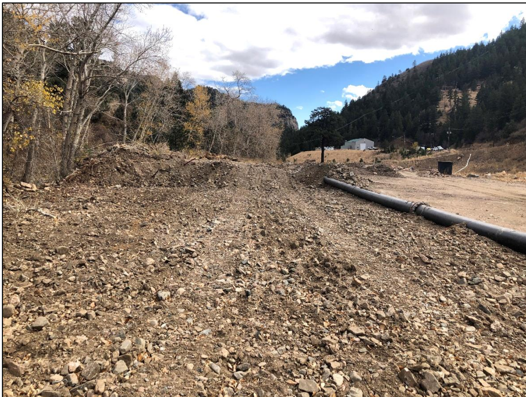
Photo 4. View looking southeast across recent excavation area along western edge of creek channel (in northwestern project area). Note bypass pipeline (at right) temporarily relocated.
