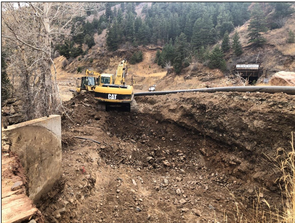
Photo 6. Closer view of current excavation activities (in northwestern project area) adjacent to southeastern toe of SWRP (and bridge access to storage area north of creek; portion of bridge visible at bottom, left).
