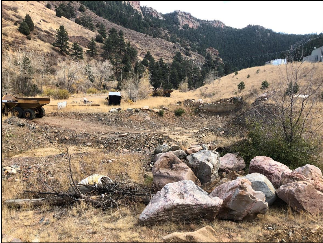
Photo 9. View looking southeast across excavation area (in northwestern project area) at toe of mesa with water treatment plant.
