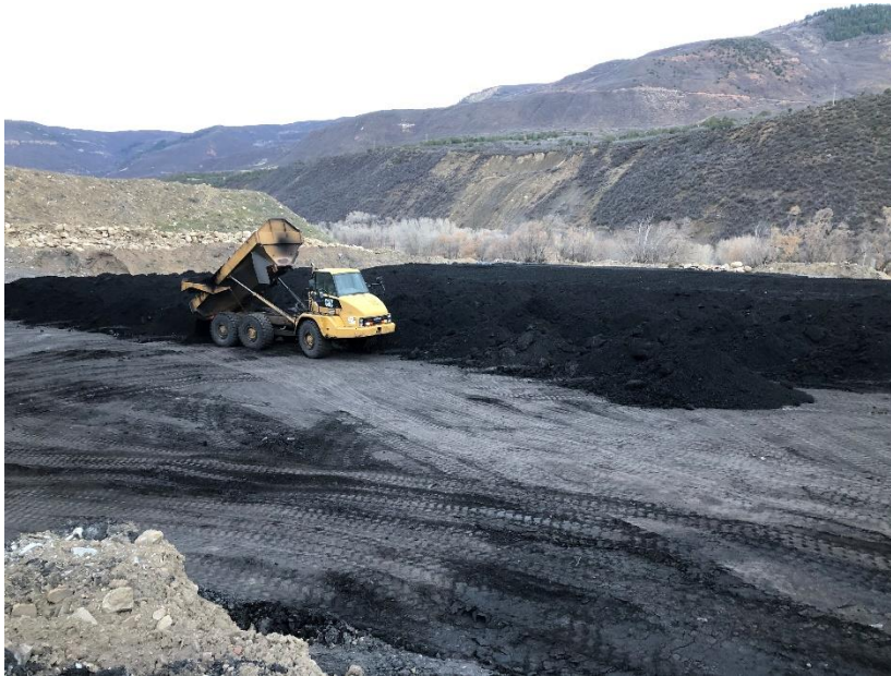
Material dumping on Gob Pile #3, prior to spreading and compacting
