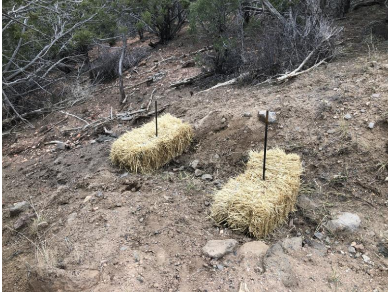
Newly installed straw bales southeast of RDA
