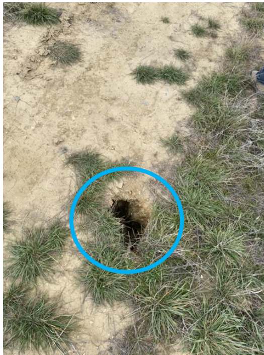
Photo 4: The hole or burrow on top of the Last Chance Pond's embankment outlined by the blue circle.
