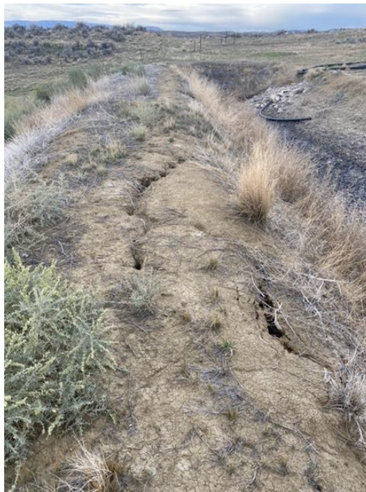
Photo 2: The cracks on top of the embankment of B Seam Dewatering System's 1 st cell.
