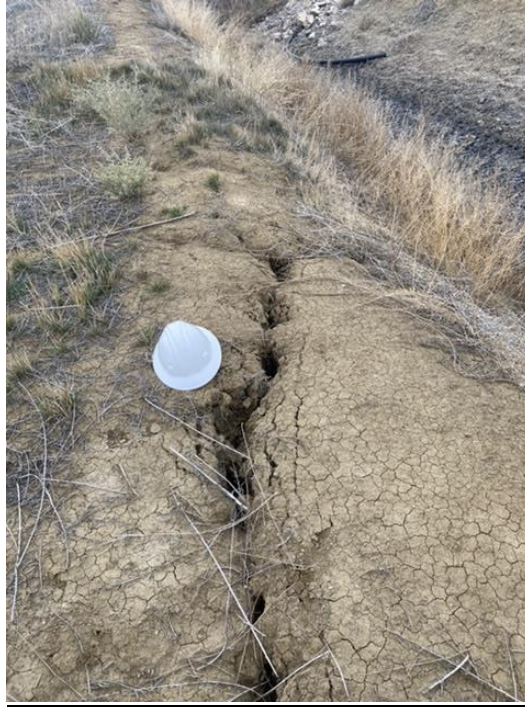
Photo 3: A hardhat for scale next to the cracks on top of the B Seam Dewatering System No. 2's 1 st cell.
