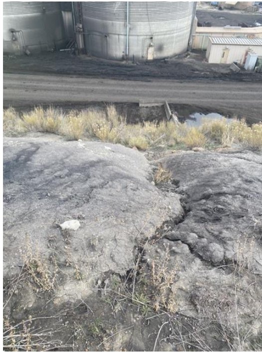
Photo 10: The rills on the slope between the upper and middle benches at the Main Facilities/Portals Area.
