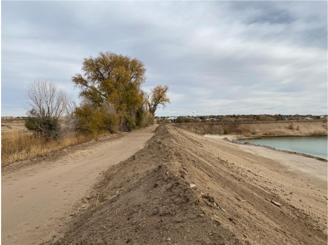
Photo 5. Stockpiled sand for final lift, access road and ditch (looking east)
