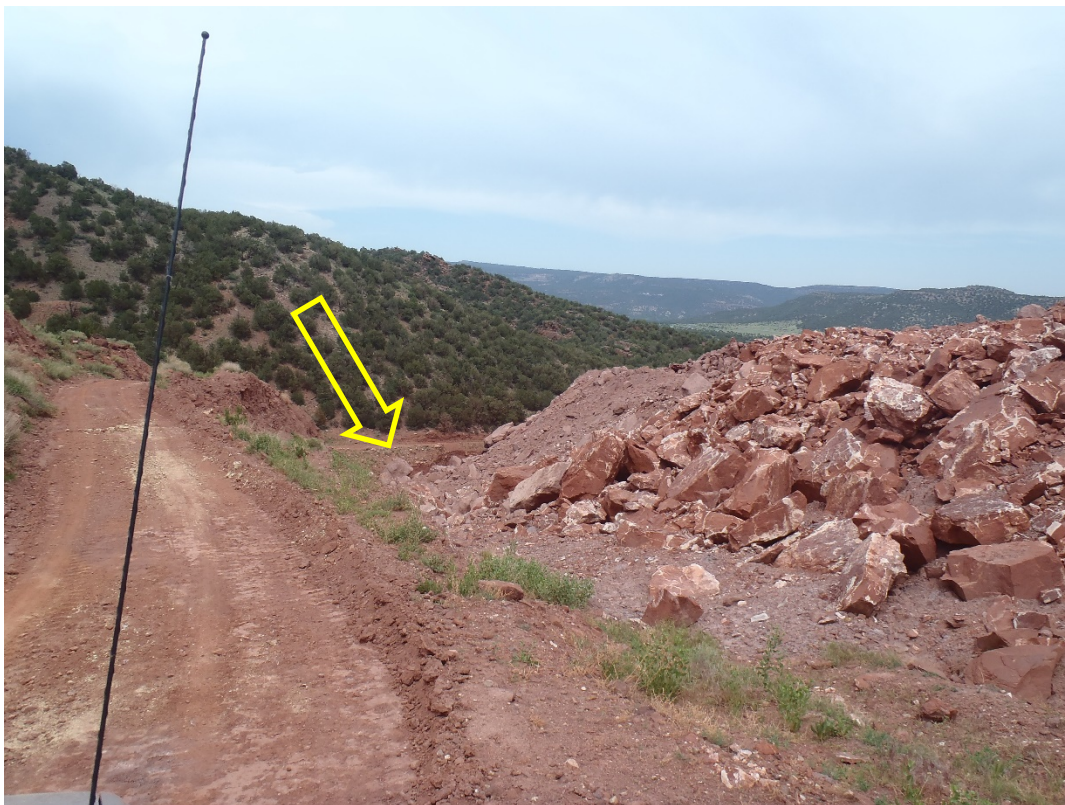
Photo 1. Backfill in gully between access road and working bench (a.k.a. NW facing highwall, looking NE).
