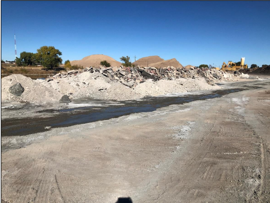
Photo 11. View looking northeast at concrete waste material piled along southern edge of Phase 1 pond to be backfilled into pond.
