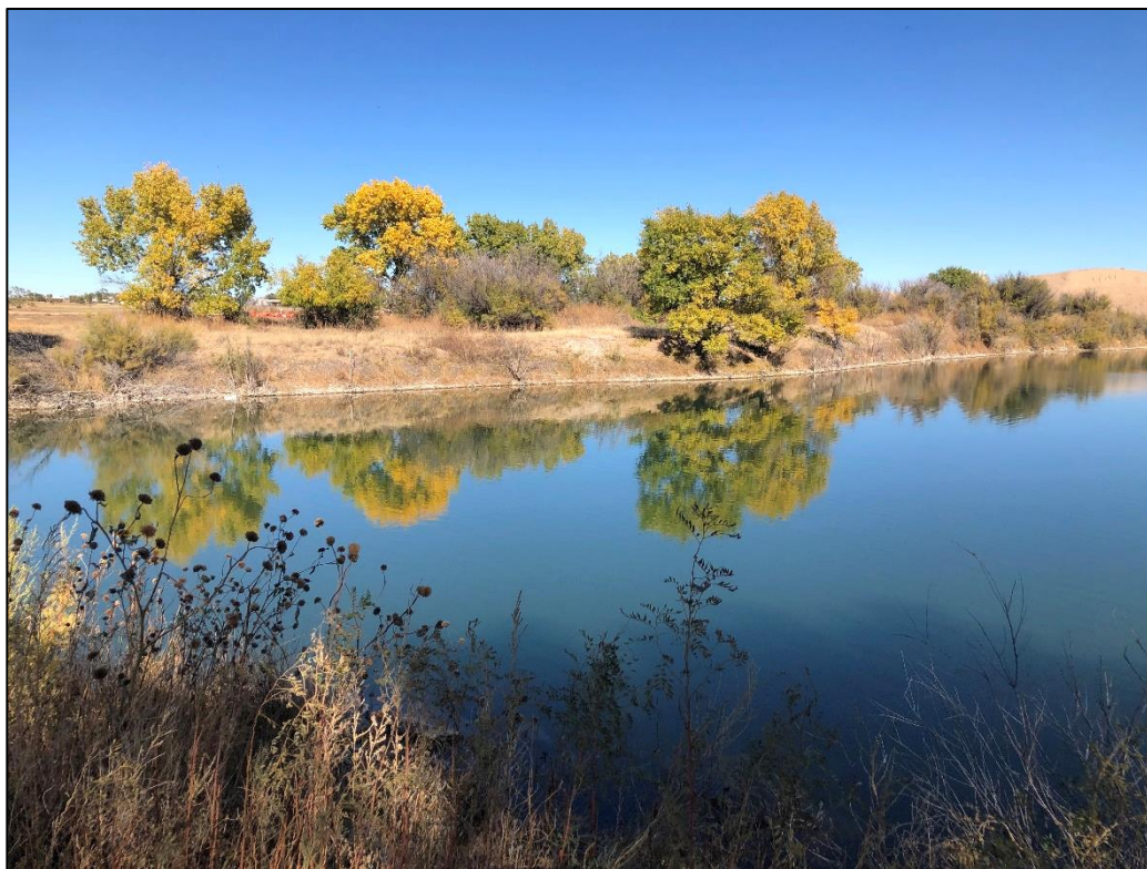
Photo 9. View looking northeast at northern shoreline of Phase 1 pond, with slopes at approximately 2H:1V. All pond slopes must be graded to 3H:1V or flatter for reclamation.
