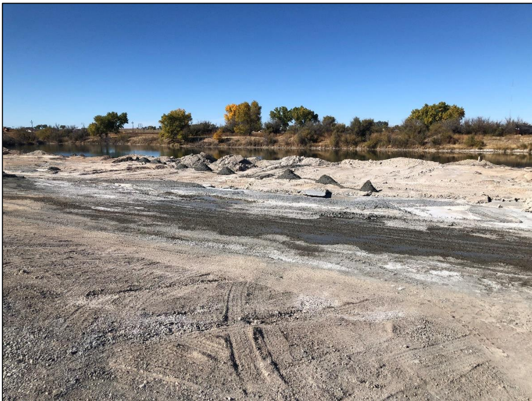
Photo 12. View looking northwest at concrete waste material piled along southern edge of Phase 1 pond to be backfilled into pond. Operator will need to specify areas where exposed concrete is present at ground surface (from previous use as wash pond) and describe how these areas will be reclaimed.
