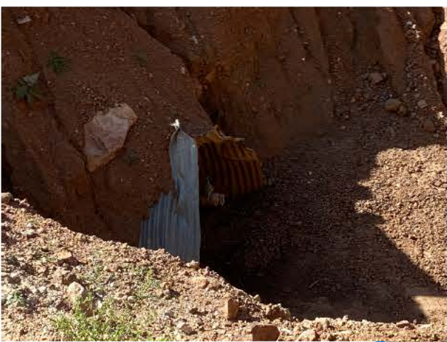
5. CULVERT INLET WITH CULVERT JETTER INSIDE
