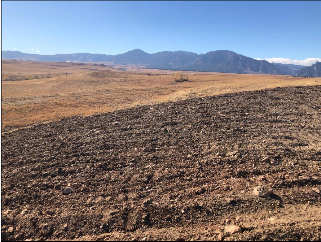
Photo 3. View looking west across southwestern side slope of upper backfill lift, graded to 3H:1V or flatter and scarified.
