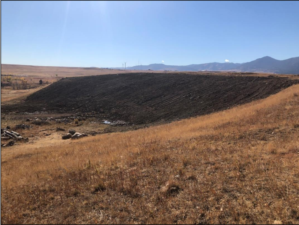
Photo 1. View looking southwest from access road at eastern side slope of lower backfill lift, graded to 3H:1V or flatter and scarified.
