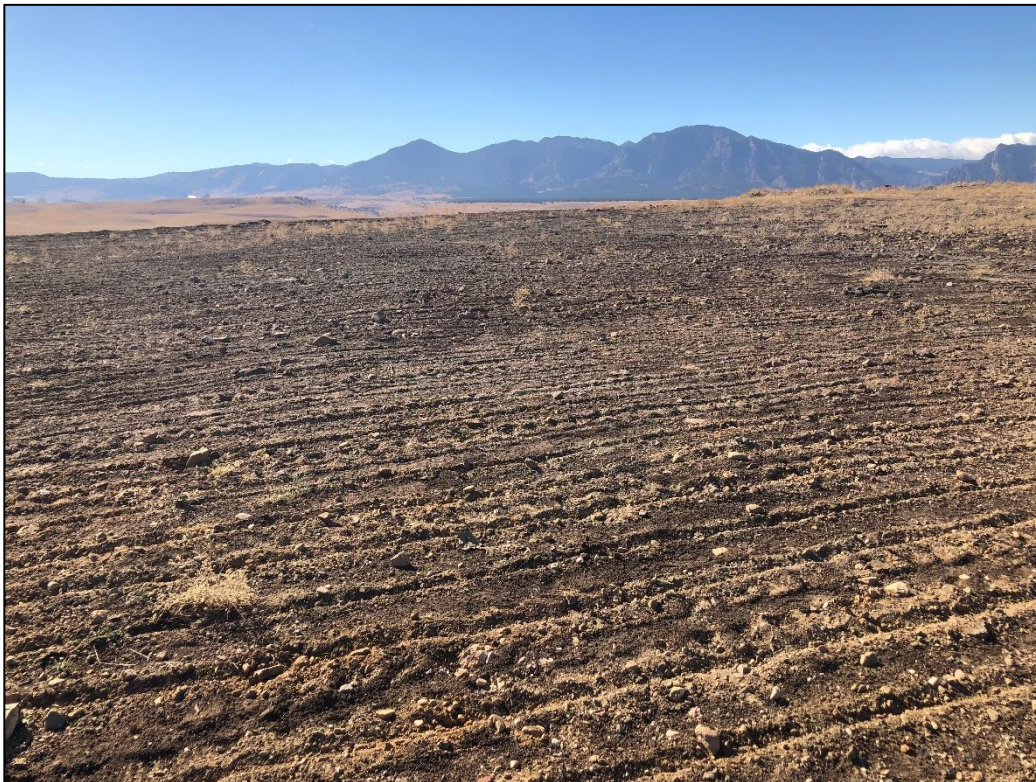
Photo 2. View looking southwest across top of upper backfill lift graded nearly flat and scarified.
