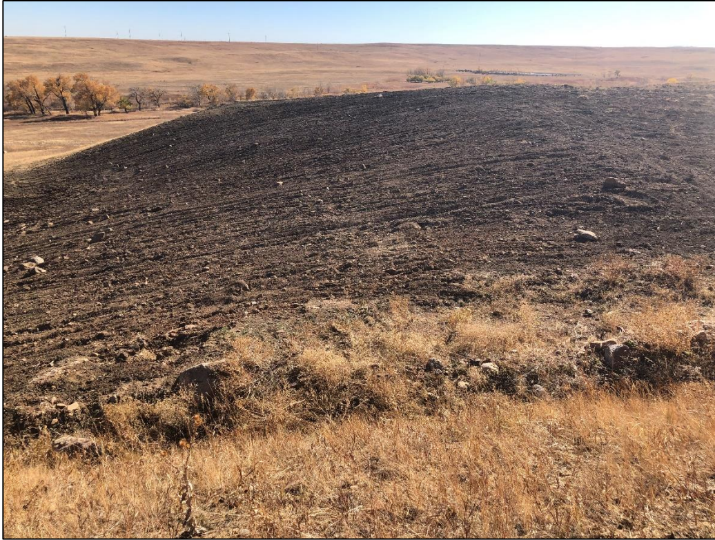
Photo 7. View looking south across eastern side slope of lower backfill lift, graded to 3H:1V or flatter and scarified.
