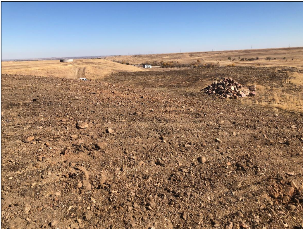
Photo 4. View looking east across southeastern side slope of upper backfill lift, graded to 3H:1V or flatter and scarified. Note small pile of boulders (on top of lower lift) to be removed from the site.
