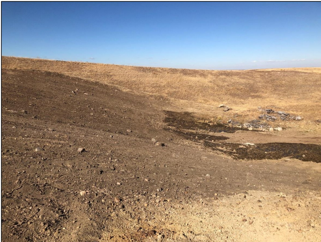
Photo 10. View looking north across eastern side slope of lower backfill lift, graded to 3H:1V or flatter and scarified. Note small seepage area at toe of lift (at left) which may require additional backfill to mitigate.
