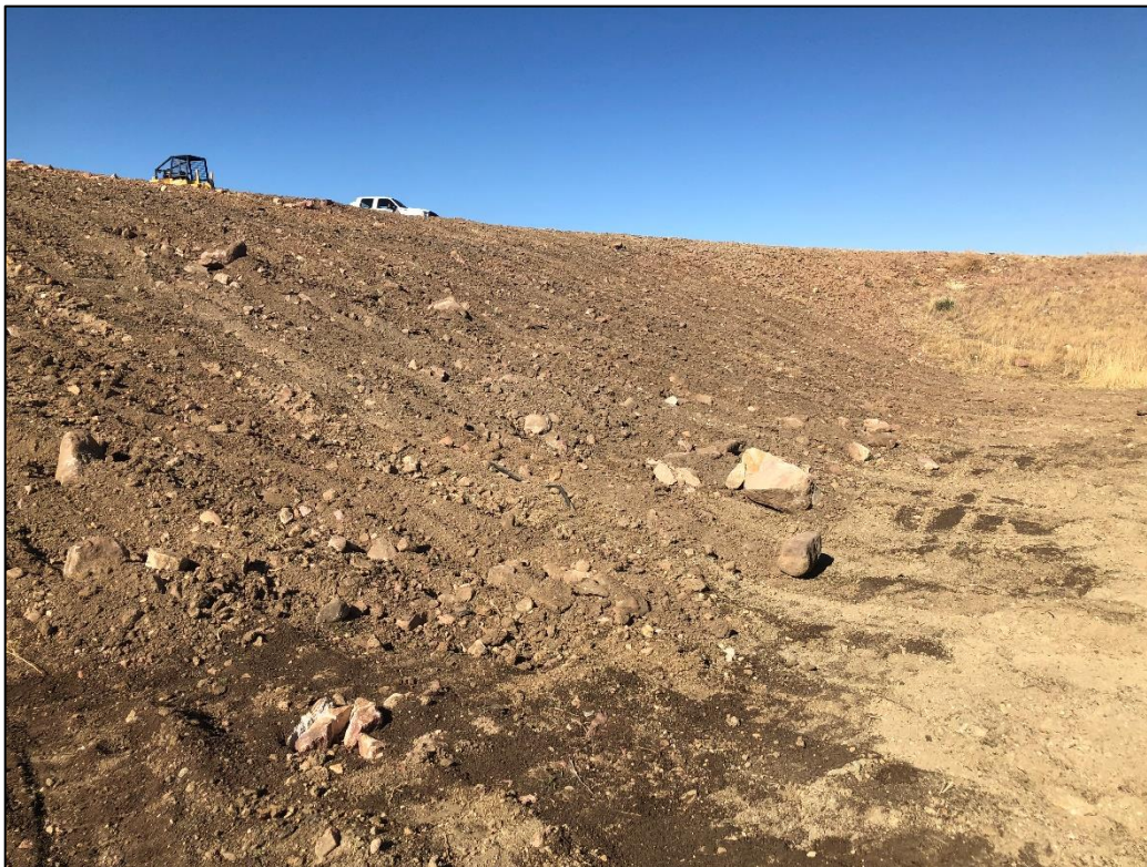
Photo 6. View looking north across eastern side slope of upper backfill lift, graded to 3H:1V or flatter and scarified.
