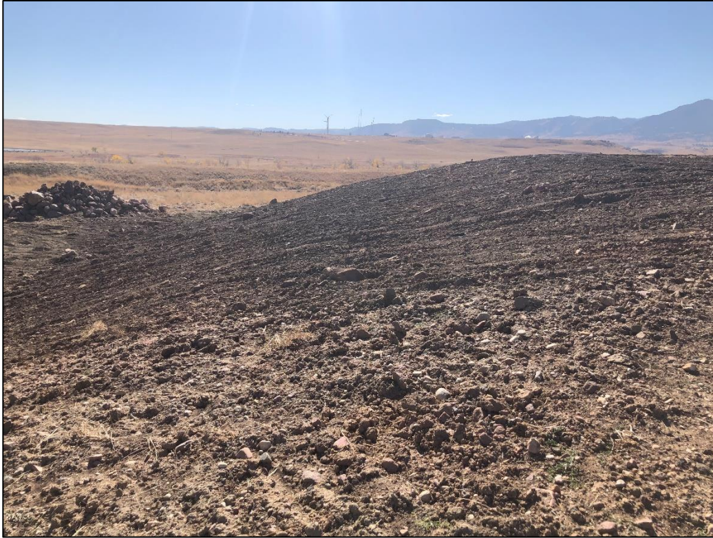
Photo 5. View looking south across eastern side slope of upper backfill lift, graded to 3H:1V or flatter and scarified.
