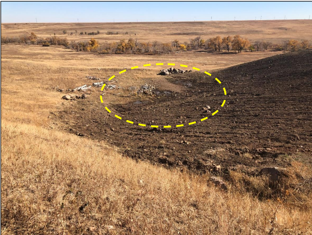
Photo 8. View looking southeast at eastern toe of lower backfill lift, showing small seepage area (circled) which may require additional backfill to mitigate.
