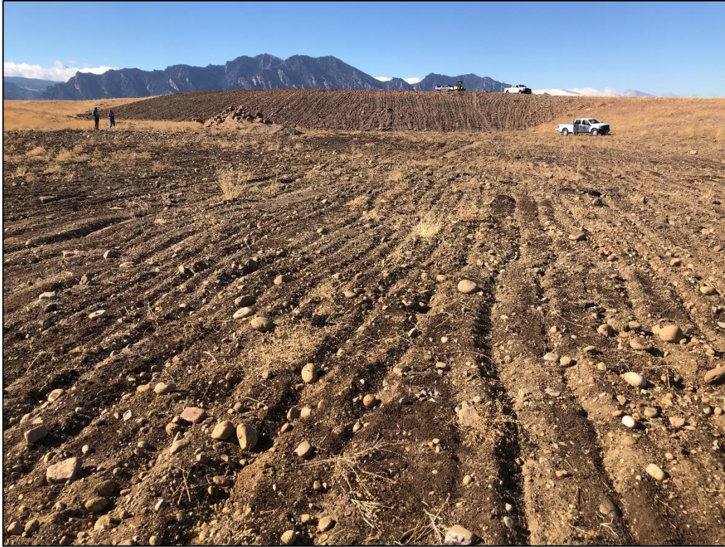
Photo 9. View looking west across top of lower backfill lift graded nearly flat and scarified. Eastern side slope of upper backfill lift visible in background.
