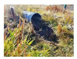
• The outlet of the discharge culvert below the Pecoco pond needs to be cleared out. It appears that this was cleaning out since the inspection in September and is full again. This may be from a previous or current beaver dam.
