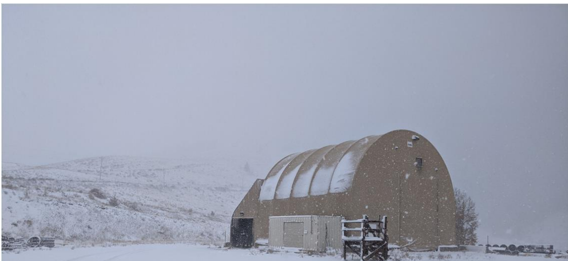
Photo One: View northeast, showing the maintenance shop located at the facilities area. The shop is in excellent condition, despite the semi-permanent building nearing the end of its design life.
