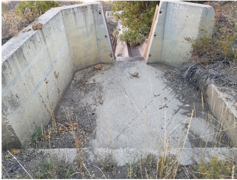
Figure 3. Upper drop down structure and flume from the end of ditch D26.
