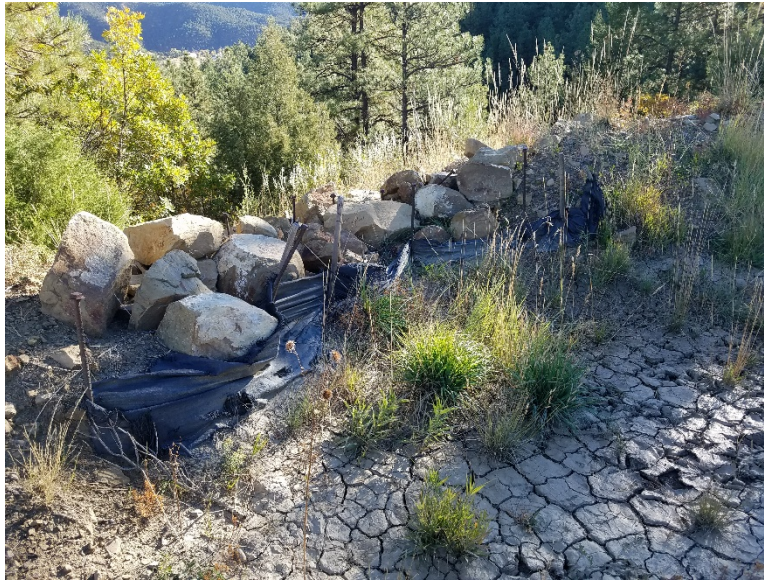
Figure 5. Drainage control structure on the pad where the water tank S.A.E. is located.
