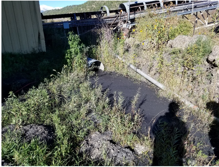
Figure 9. Culvert C64 outlet that needs to be cleaned out.
