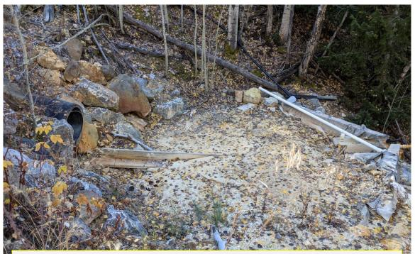
Photo Five: View south, showing the discharge sump located downgradient from the 6 level portal area in Deadman Gulch. The sump receives discharge water from the treatment system and rerouted water from Deadman gulch, where it mixes prior to discharge. The sump requires immediate cleanout prior to resumption of water treatment operations.
