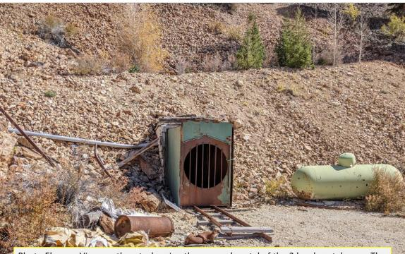
Photo Eleven: View northeast, showing the secured portal of the 3 level portal area. The portal closure is secure, and shows no signs of vandalism or attempted unauthorized entry. This portal is no longer used for operations and primarily serves as ventilation and secondary egress.
