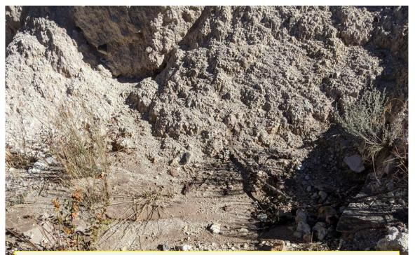
Photo Six: View northeast, showing what should be a storm water culvert inlet along the access road. The inlet has become plugged, impeding flow resulting in storm water flow from the access road reporting to the 6 level pad area. The obstructed storm water control structures require immediate repair.
