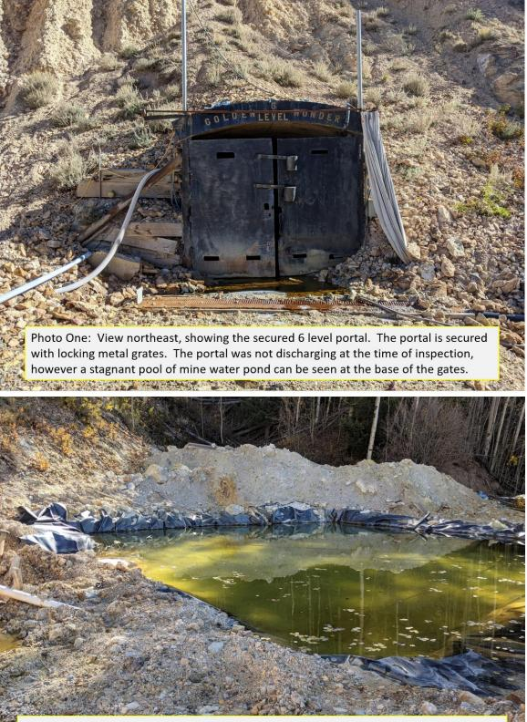
Photo Two: View southeast, showing the mine water collection pond. The pond is nearly full with minimal freeboard to account for precipitation or mine water input. The pond is lined, and the edges of the liner are secured with minimal amounts of waste rock. The pond requires immediate attention.
