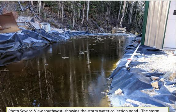
Photo Seven: View southwest, showing the storm water collection pond. The storm water pond is lined with an HDPE liner and is at maximum capacity. Almost no freeboard exists to account for additional storm water input and will result in discharge. The pond requires immediate attention.
