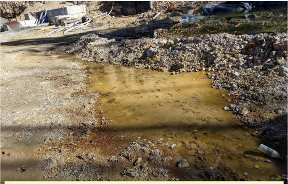
Photo Three: View north, showing the preferential flow path that the mine water discharge has established as a result of the plugged conveyance pipe that would deliver the mine water to the collection pond. Visible evidence of impaired water quality was observed.
