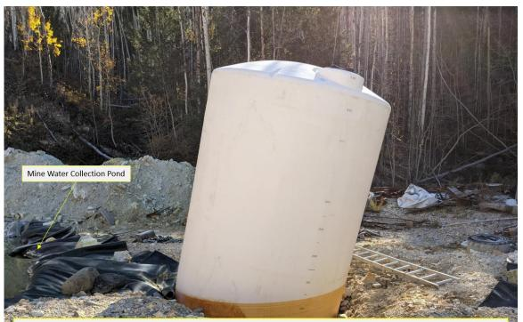
Photo Four: View southeast, showing the mine water treatment tank. The tank is located adjacent to the mine water collection pond and not set on a sound foundation. The tank and water treatment system requires immediate repair, including a proper foundation prior to the resumption of water treatment operations.
