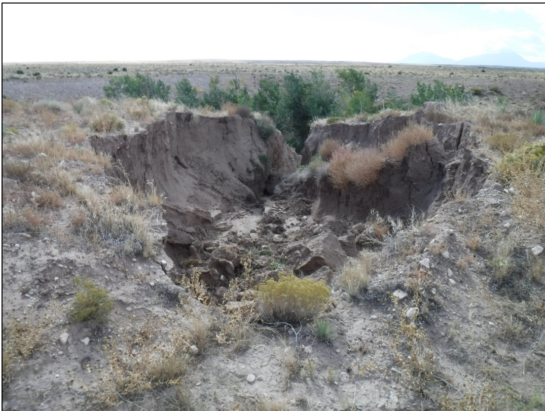
Photo 16: Headcutting of erosion gully leading to eastern pit area
