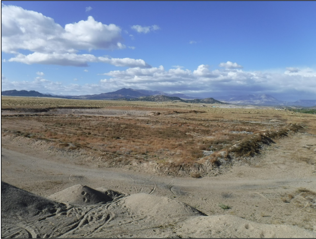
Photo 5: Previous pit area that has been backfilled
