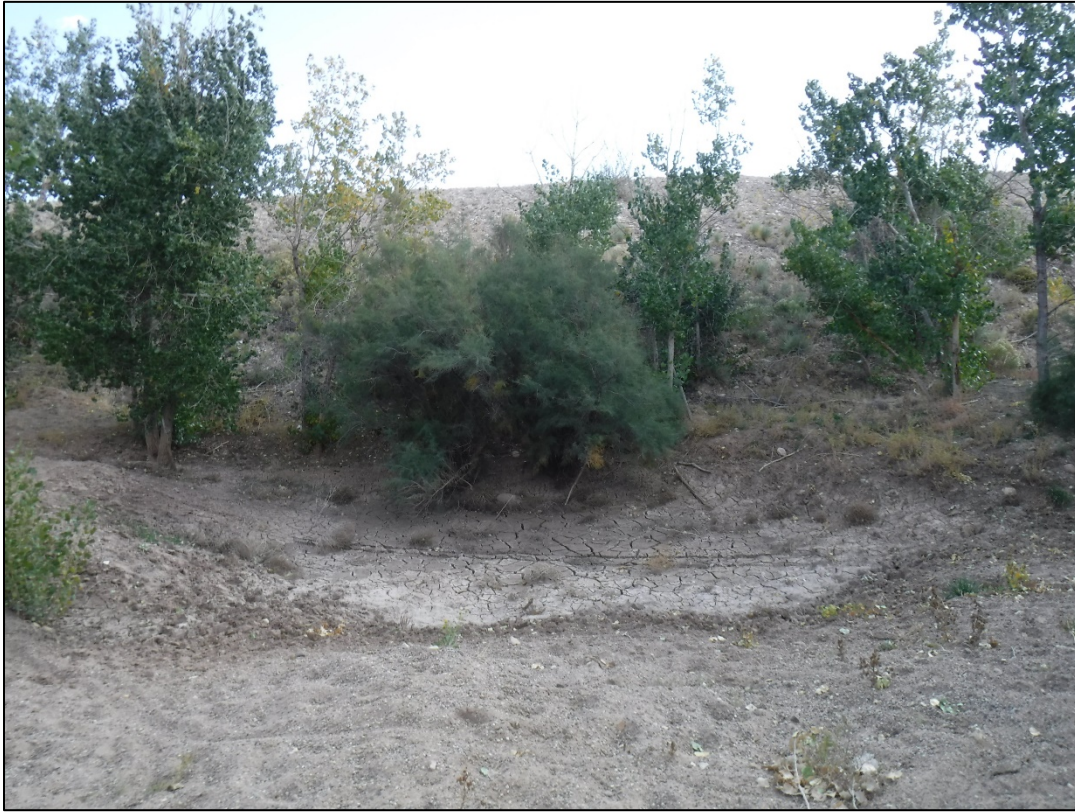
Photo 15: Saltcedar eastern pit area
