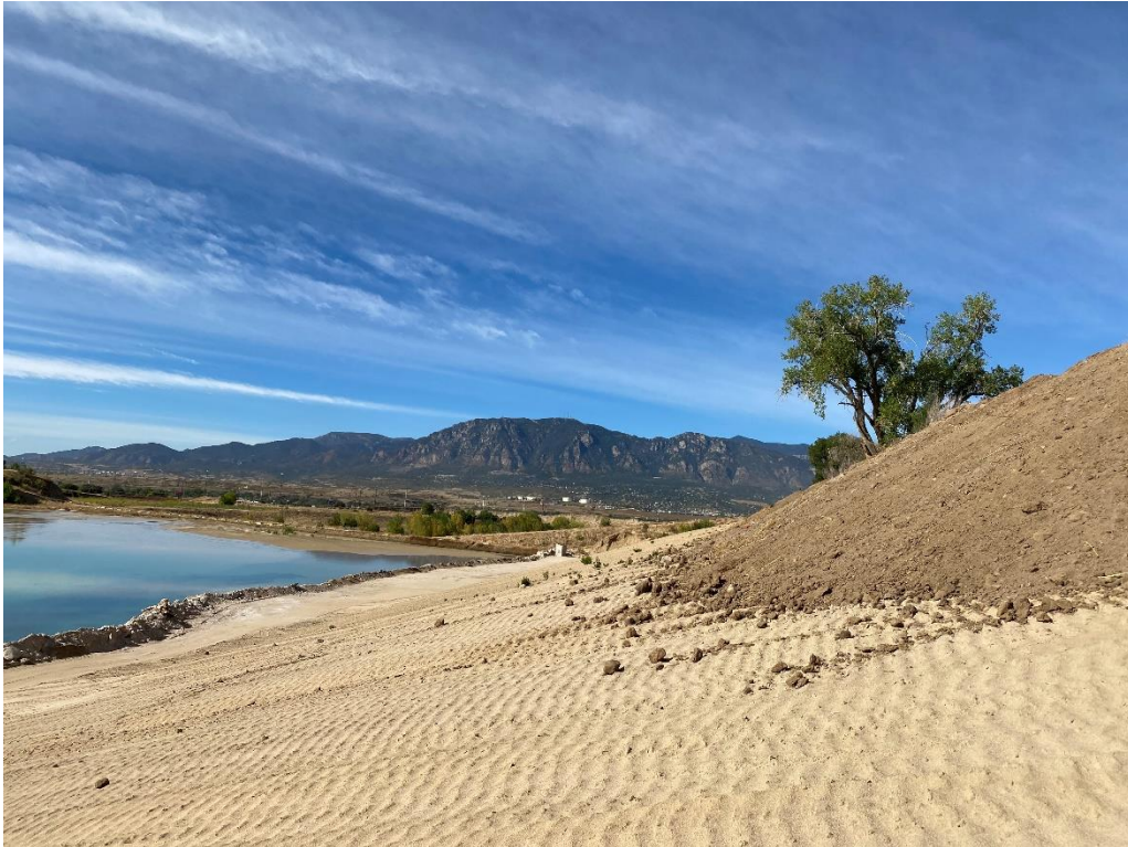
Photo 6. Stockpiled sand for final lift
