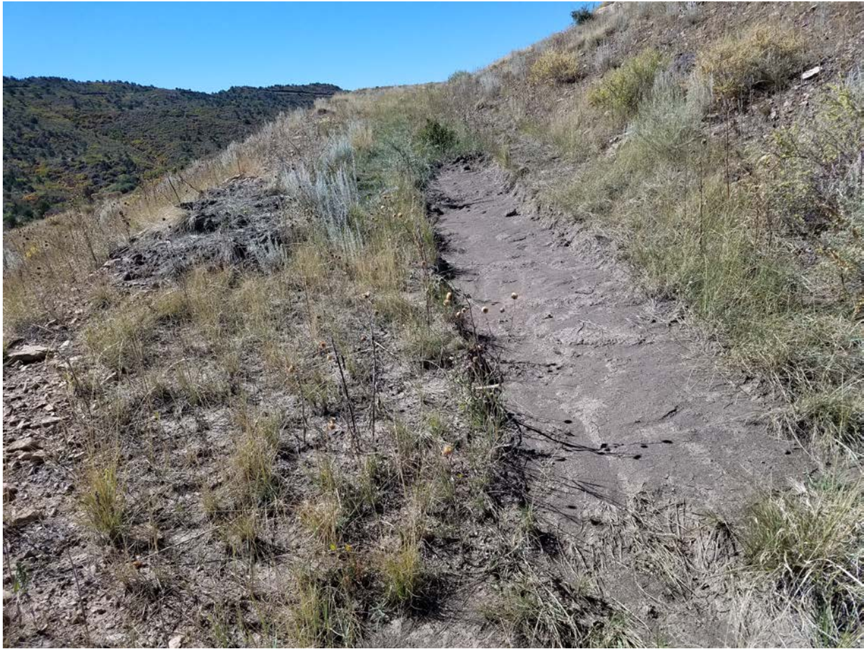
Figure 8. Repair work conducted on Fill 9 terrace and drainage ditch. Out slope repaired and positive drainage re-established to D92.
