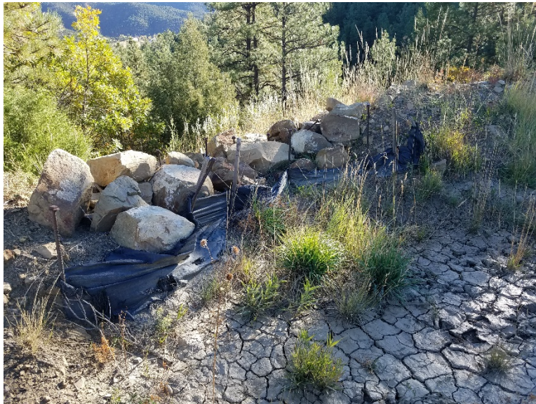
Figure 4. Drainage control structure on the pad where the water tank S.A.E. is located.
