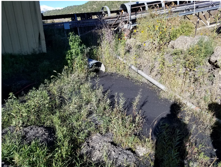
Figure 8. Culvert C64 outlet that needs to be cleaned out.
