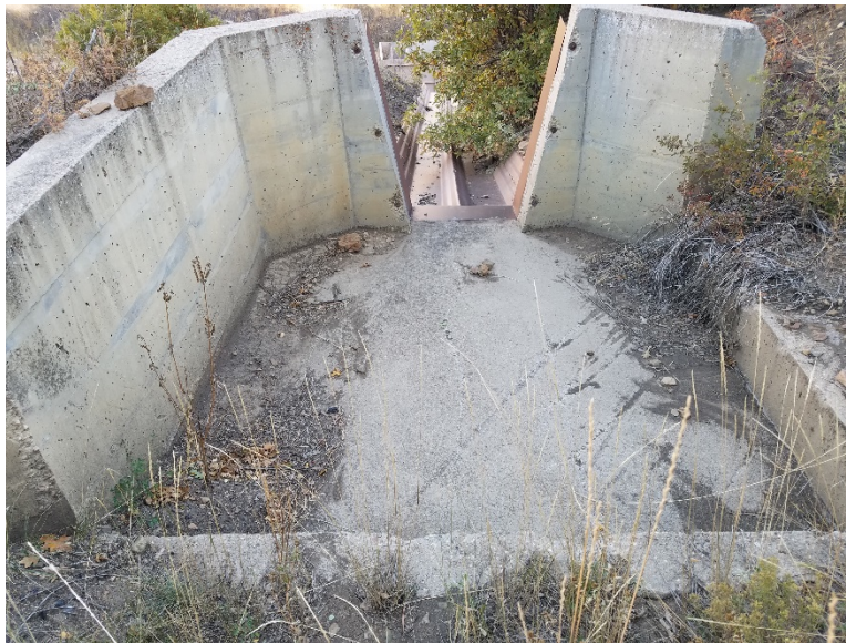
Figure 2. Upper drop down structure and flume from the end of ditch D26.
