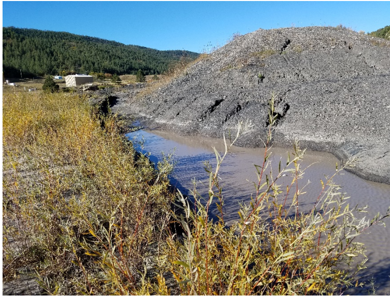
Figure 7. Sump upstream of Culvert C13 deepened.
