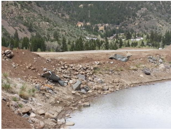
Photo 5. Debris and rock buried in pond.
