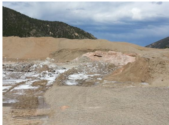
Photo 4. Salt buried onsite in 2013.
