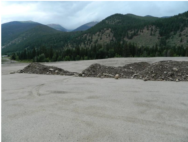
Photo 6. Imported topsoil on graded surface
