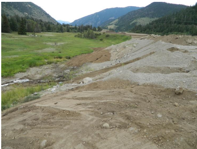
Photo 8. Topsoil spread on the prepared surface.
