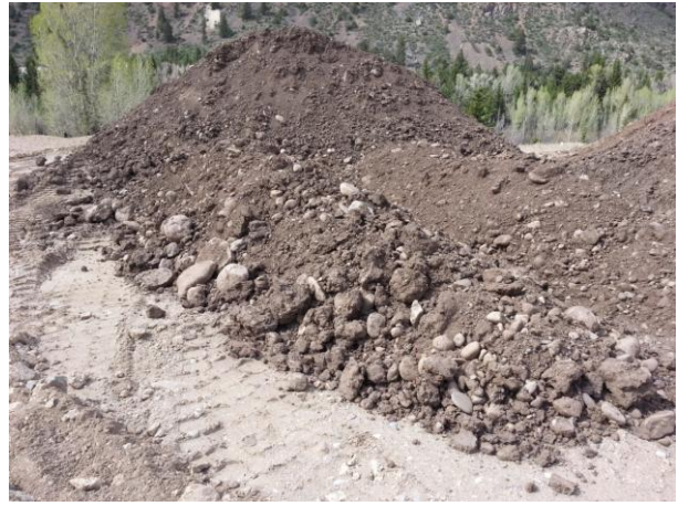
Photo 6. Imported topsoil used to cover dirt.
