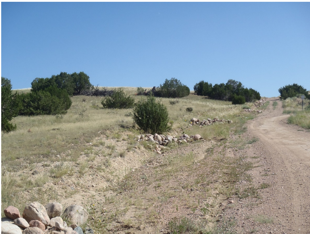
Photo 3. Access road and roadside ditch (note rock check dams).
