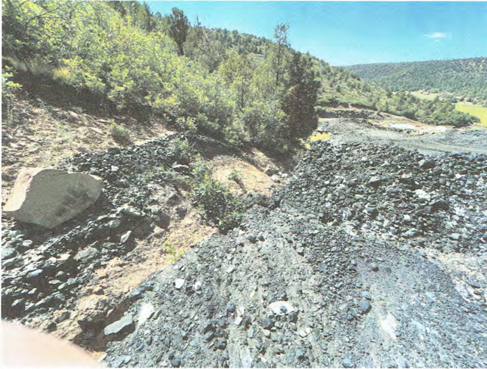
Pic. 3 – Erosion at SW corner of main waste pile at top.
