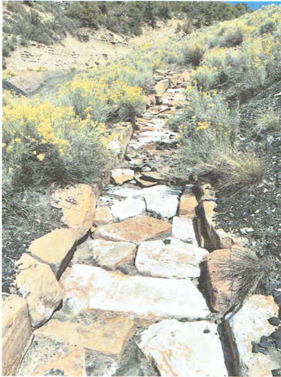
Pic. 1 –Reach 10 treated water channel in good condition.
