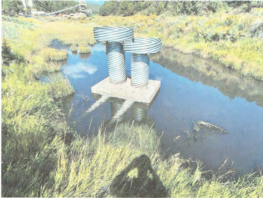
Pic. 1 – Detention Pond outlet in good condition.
