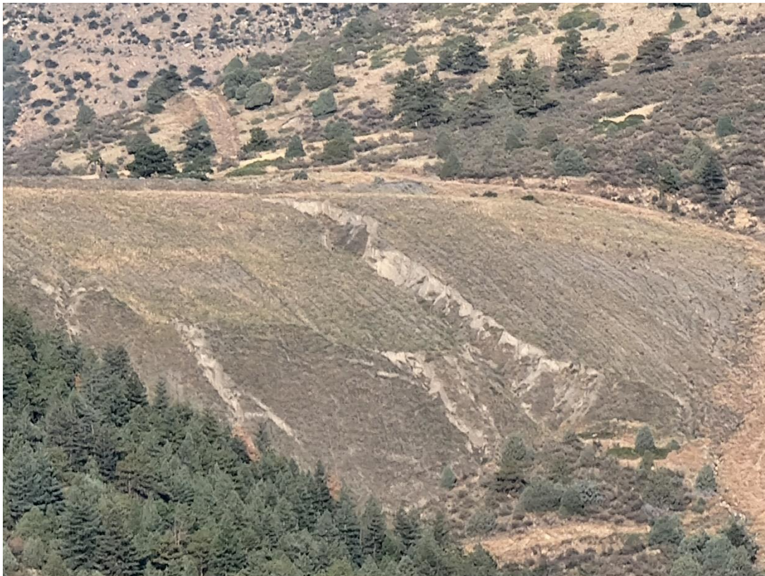
(A.) Frei's Gilpin Waste Fines Dump erosion visible from the northeast
