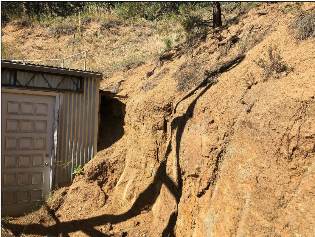
Photo 8. View looking southwest across steep northern slope adjacent to winch house. This slope must be graded to 3H:1V for reclamation. Steeper bedrock slopes behind winch house may remain if reclamation plan is revised to leave winch house and steeper slopes in this area.
