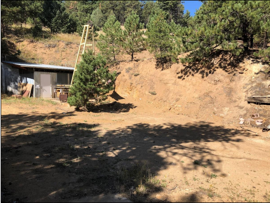
Photo 7. View looking northwest at northern slope of mining area which must be graded to 3H:1V for reclamation.
