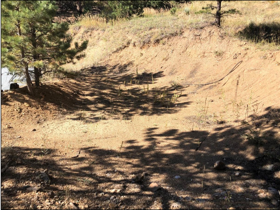
Photo 3. View looking southwest across leveled area on hillside W/NW of mining area which was used for stockpile storage. This area must be graded to 3H:1V, retopsoiled, and revegetated for reclamation.
