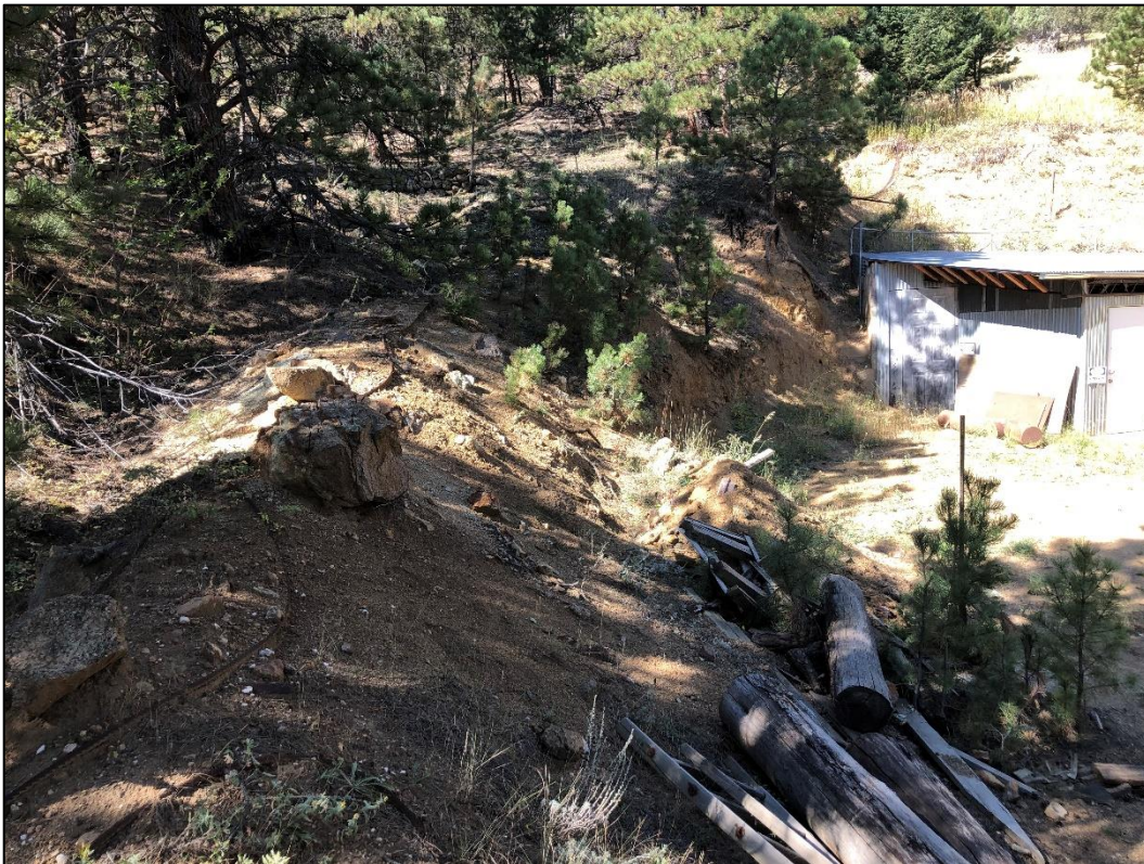
Photo 6. View looking southwest across southern slope of mining area. This slope must be graded to 3H:1V for reclamation. Steeper bedrock slopes behind winch house (at right) may remain if reclamation plan is revised to leave winch house and steeper slopes in this area.
