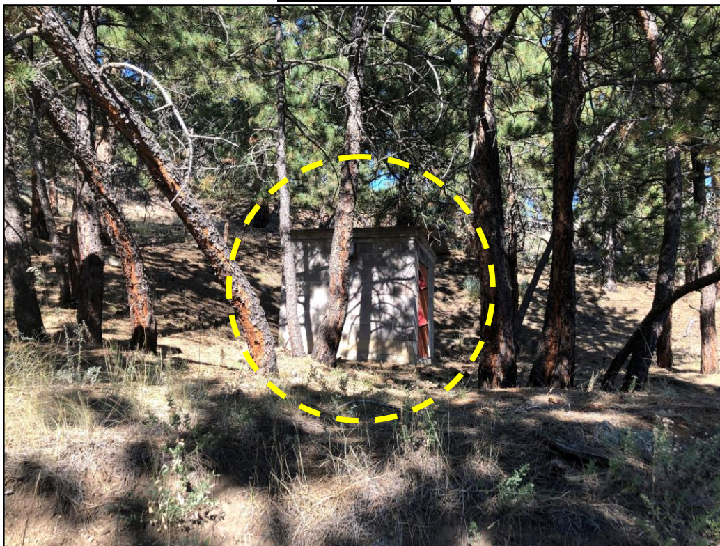
Photo 1. View looking north at (empty) powder storage building (circled) located W/NW of mining area. This building will remain for reclamation.
