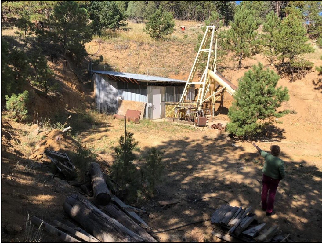
Photo 5. View looking southwest across mining area, showing winch house and headframe which must be removed, unless reclamation plan is revised to leave winch house (headframe must be removed). Steep slopes encircling this area must be graded to 3H:1V, and the area retopsoiled and revegetated for reclamation.
