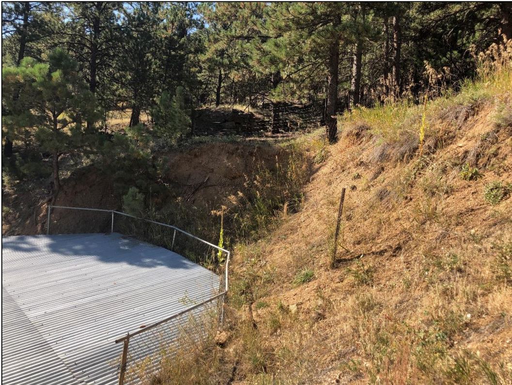
Photo 4. View looking southwest across steep slope behind winch house (roof of winch house visible at bottom, left). This slope must be graded to 3H:1V, unless reclamation plan is revised to leave winch house and steeper slopes in this area.
