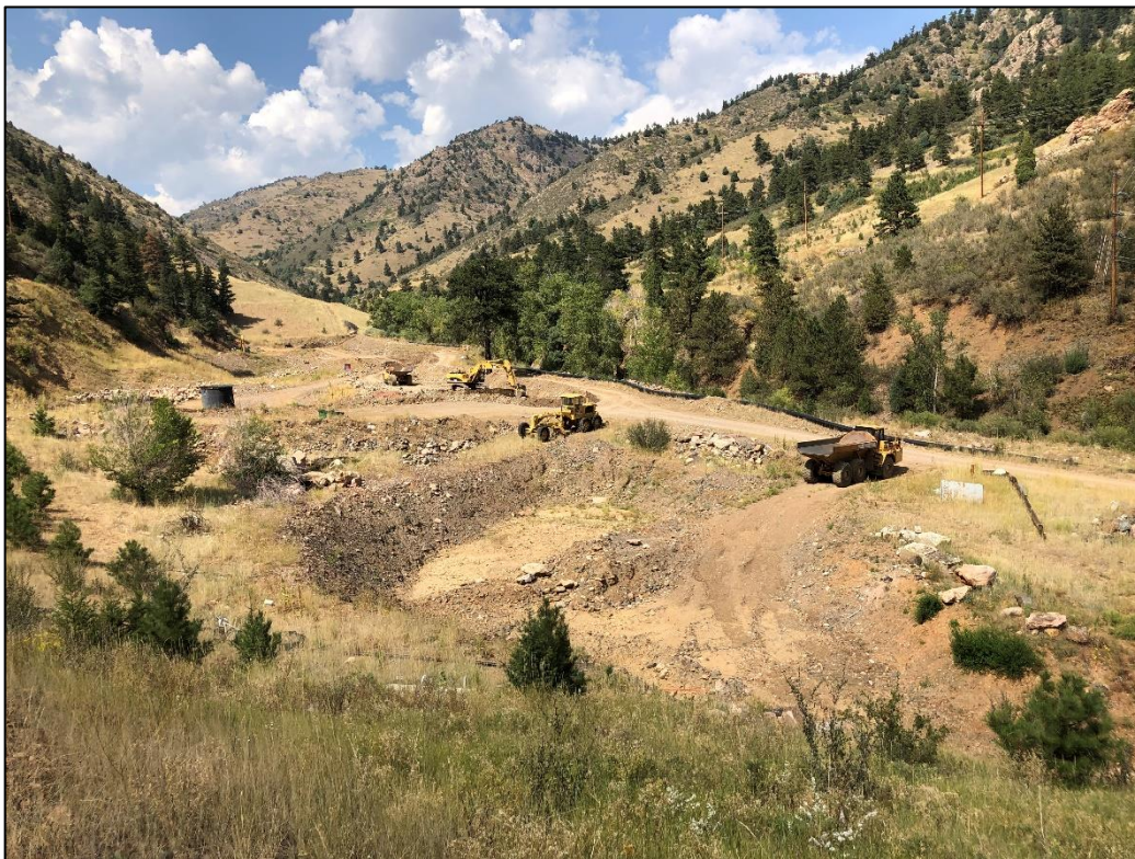
Photo 4. View looking northwest (from top of mesa with water treatment plant) across northern portion of valley excavation project, in which, excavation activities were occurring during inspection. Radionuclide-impacted alluvial valley soils are excavated and disposed of underground per the approved permit.
