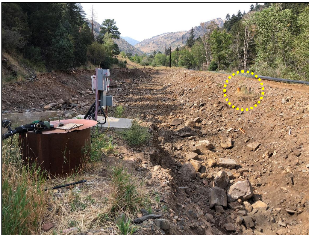
Photo 11. View looking northwest across southern portion of valley excavation project. Note alluvial groundwater monitoring well MW-7 (circled) which operator may propose (in an upcoming Technical Revision) to abandon, since alluvial material surrounding well must be removed for valley excavation project. Sump #1 (at left; the last functional sump on site) may also become redundant.
