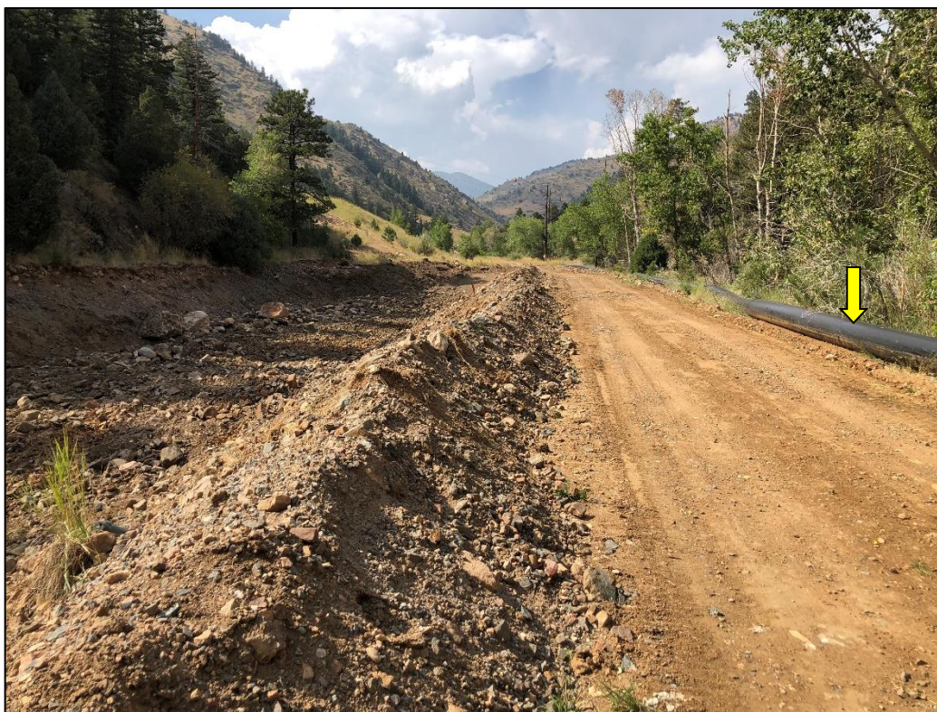
Photo 10. View looking northwest across southern portion of valley excavation project, showing recent excavation along south side of access road. Road and adjacent bypass pipeline (indicated) may need to be temporarily relocated during this project.
