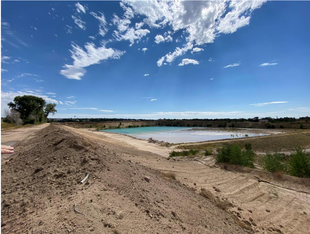
Photo 4. Stockpiled sand for final lift
