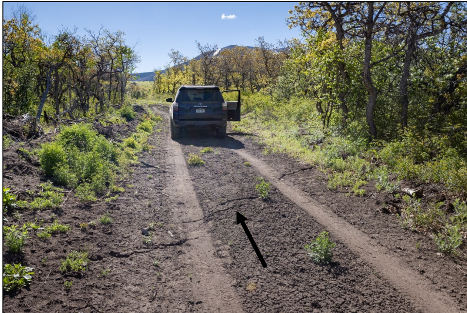
Figure 9. Northwestward view during the spring 2021 field visit of a subsidence crack first observed during our spring 2019 field visit. The 6-inch elevation offset from north to south (right to left) is still present, but materials have filled the deepest portions of the crack and rounded the edges. This location is approximately 1,000 feet north of the MVB E6-14 pad.
