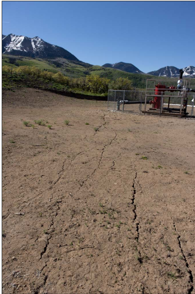
Figure 10. Southeastward view during the spring 2021 field visit of a group of sub-parallel cracks on the northwest portion of the MVB SS1-7 pad. Longwall mining had recently passed beneath this area.
