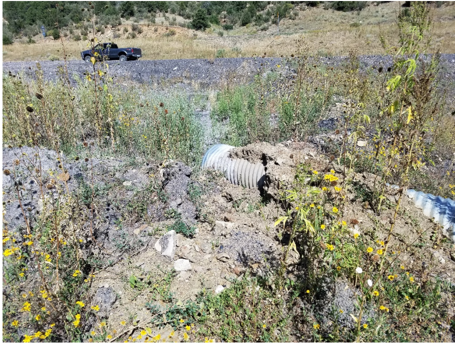
Figure 5. Berm directing flow to culver C-13 breached and needs repair.
