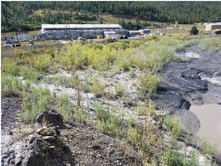
Figure 4. DWDA #2, southeast corner. Sump where D14 and D12 meet at culver C13. This area needs to be cleaned out.
