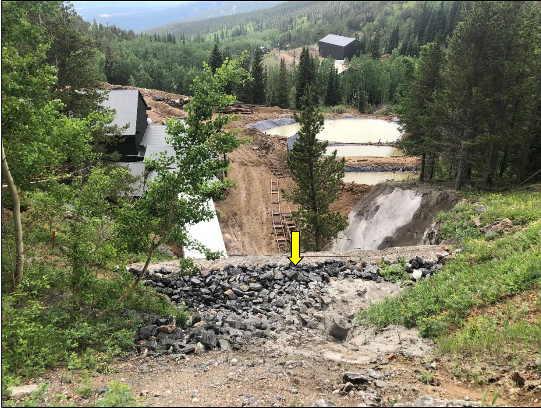
Photo 31. View looking southeast from Caribou Road across slope above Idaho Tunnel Portal where small “glory hole” created by tunnel collapse (location indicated) was stabilized with pervious cellular concrete per TR-5. This disturbed slope is part of the expansion area proposed in AM-2.
