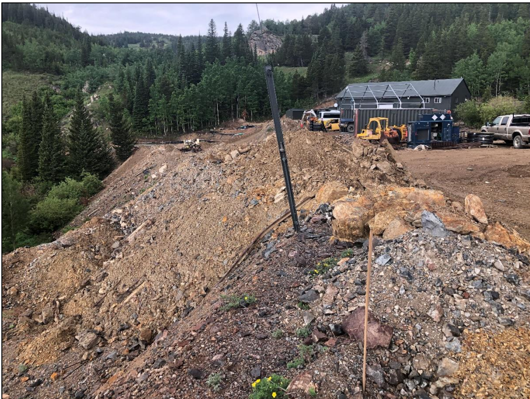
Photo 38. View looking west across southern slope of historic waste rock pile located in Caribou Mine area, with slope gradients of approximately 1H:1V.
