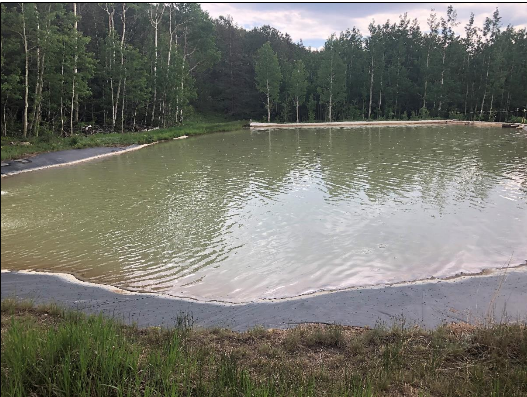
Photo 14. View looking southeast across Pond 2 in which water from each mine is combined prior to being discharged to Coon Track Creek under NPDES permit. Operator should remove any sediment or vegetation from pond liner to maintain adequate freeboard and protect liner integrity.
