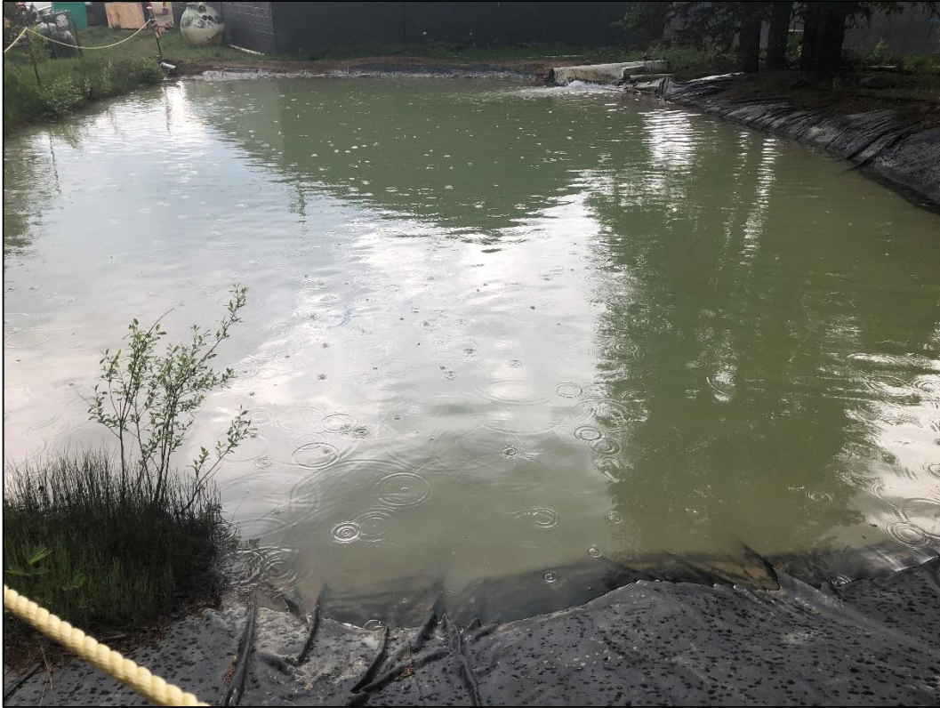
Photo 15. View looking southeast across Pond 1, in which Cross Mine water is discharged and treated with lime daily. Water from this pond gravity drains to Pond 2. Operator should remove any sediment or vegetation from pond liner to maintain adequate freeboard and protect liner integrity.
