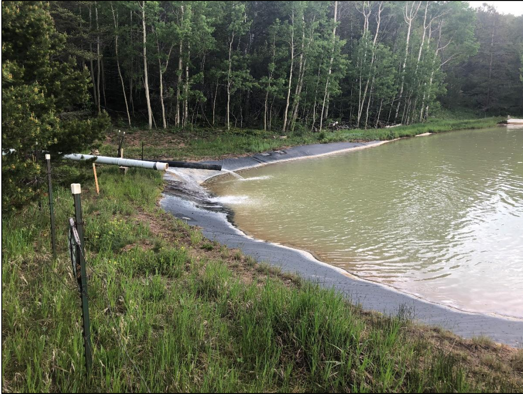
Photo 13. View looking east across northern corner of Pond 2, showing discharge into pond from Pond 1 (Cross Mine; white pipeline) and Ponds 3A-3C (Caribou Mine; black pipeline). The proposed expansion area in AM-2 would include the northern edge of this pond with the discharge pipelines.
