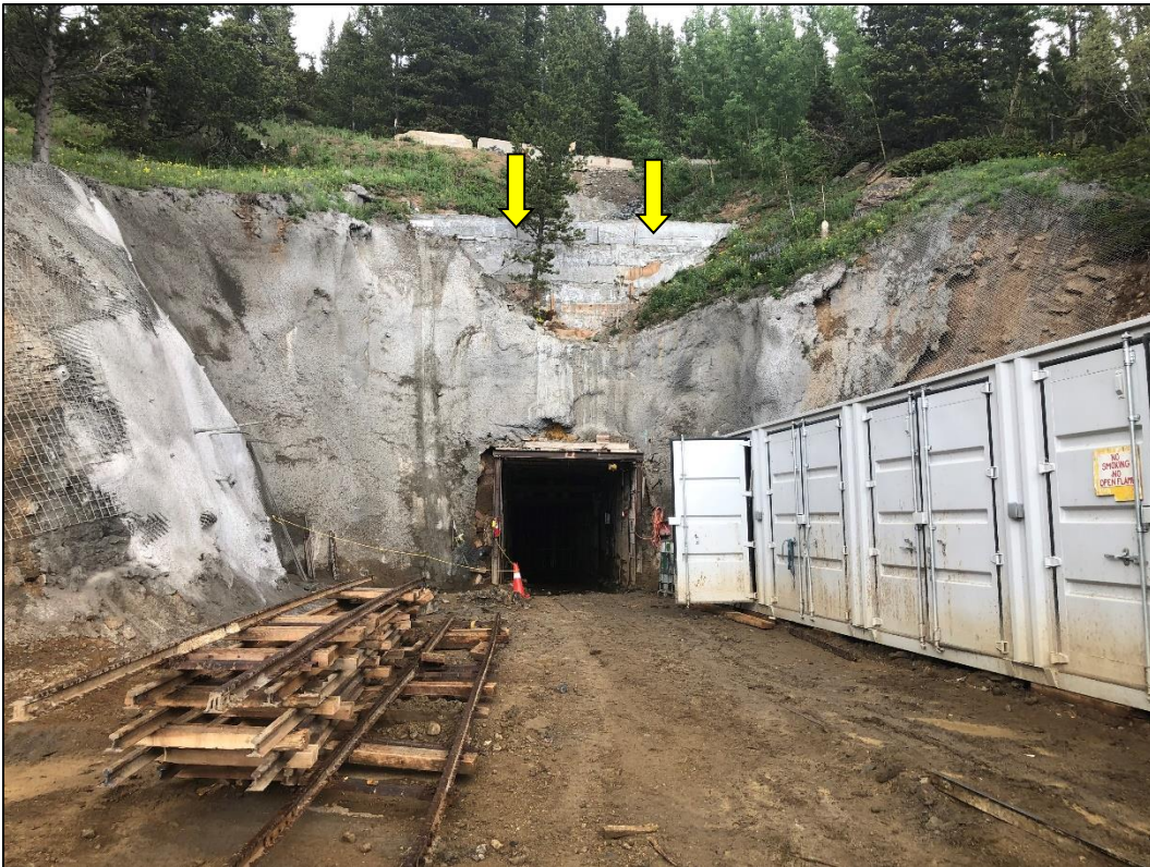
Photo 28. View looking northwest at expansion area proposed in AM-2 with Idaho Tunnel portal (in Caribou Mine area). Note surrounding slope face stabilized with shotcrete and small “glory hole” created by tunnel collapse (location indicated) stabilized with pervious cellular concrete per TR-5.
