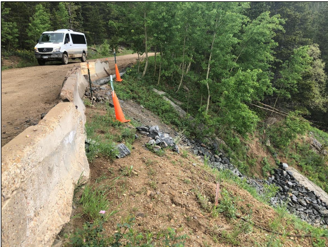
Photo 32. View looking northeast across slope between Caribou Road (at left) and area above Idaho Tunnel Portal (at right) where small “glory hole” was stabilized with pervious cellular concrete per TR-5. This disturbed slope is part of the expansion area proposed in AM-2. The new northern permit boundary in this area would align with the edge of Caribou Road.
