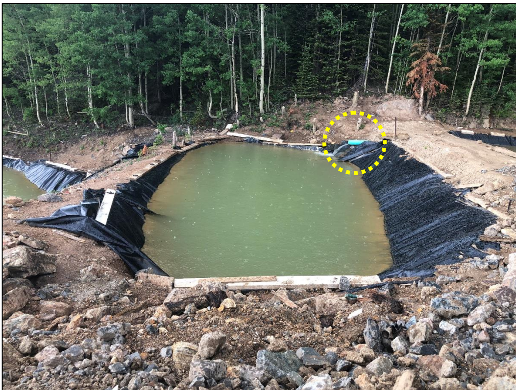
Photo 26. View looking southwest across Pond 3B (in Caribou Mine area) which was rehabilitated per TR-8. This is the middle of the three settling ponds. Note inlet pipe from Pond 3A (circled) discharging into pond.
