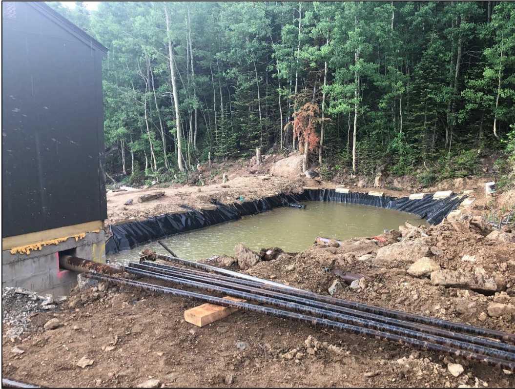
Photo 27. View looking southwest across Pond 3A (in Caribou Mine area) which was rehabilitated per TR-8. This is the most upgradient of the three settling ponds.
