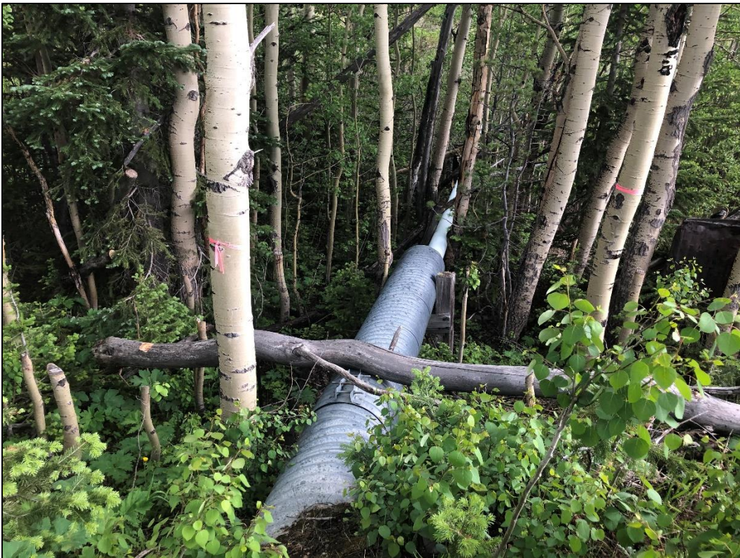
Photo 16. View looking east at drainage pipeline which conveys treated Cross Mine water from Pond 1 to Pond 2.
