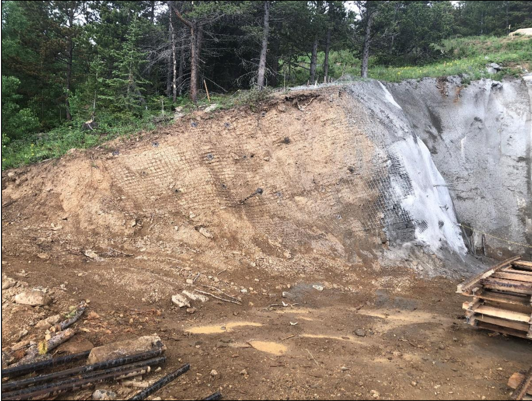
Photo 29. View looking northwest at excavated hillside just west/southwest of Idaho Tunnel Portal (in Caribou Mine area) which is part of expansion area proposed in AM-2. This slope face is stabilized partially with shotcrete and partially with wire mesh anchored into the slope.
