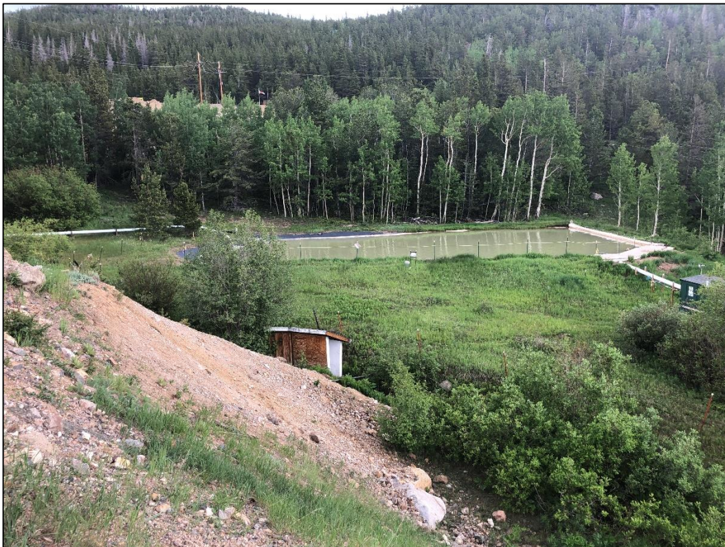
Photo 10. View looking north across valley between Cross and Caribou Mines, showing Pond 2 in which water from each mine is combined prior to being discharged to Coon Track Creek under NPDES permit.
