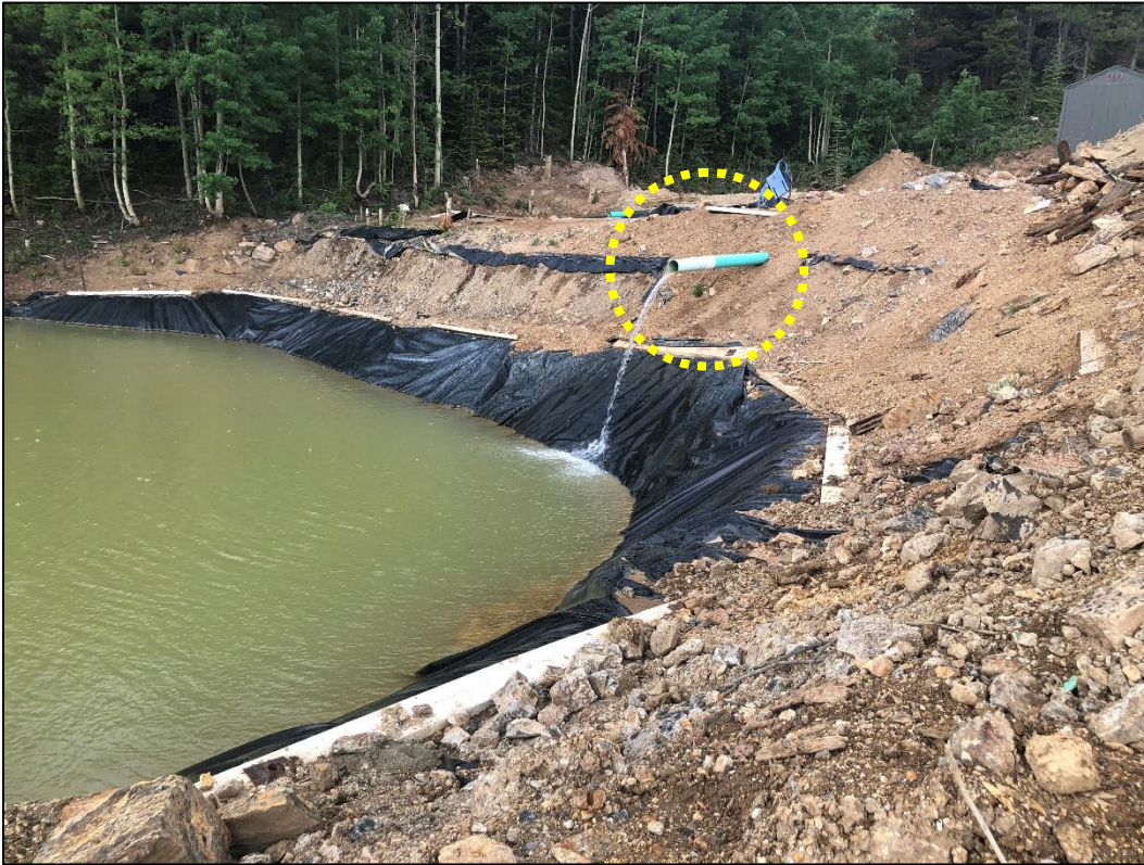
Photo 25. View looking west across northern edge of Pond 3C (in Caribou Mine area) which was rehabilitated per TR-8, showing inlet pipe from Pond 3B (circled) discharging into pond.
