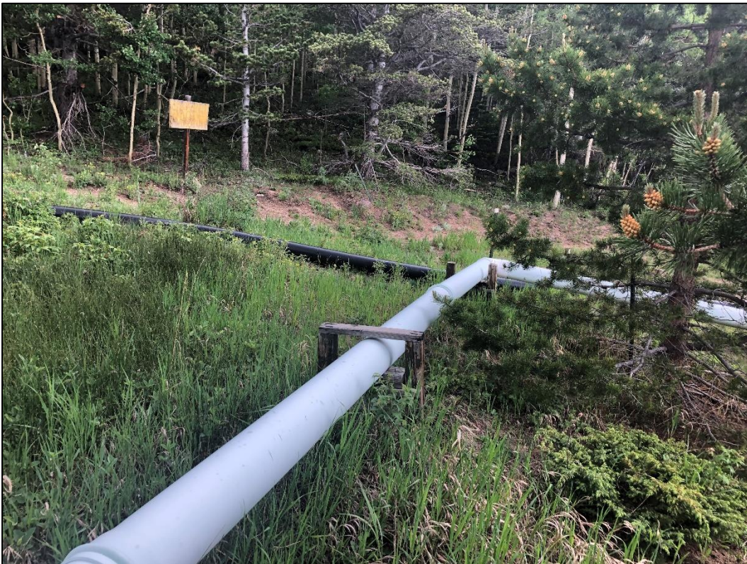
Photo 12. View looking northeast at expansion area proposed in AM-2 for pond water pipelines, located directly north of Pond 2. Note white pipeline which conveys water from Pond 1 (at Cross Mine) and black pipeline which conveys water from Ponds 3A-3C (at Caribou Mine).
