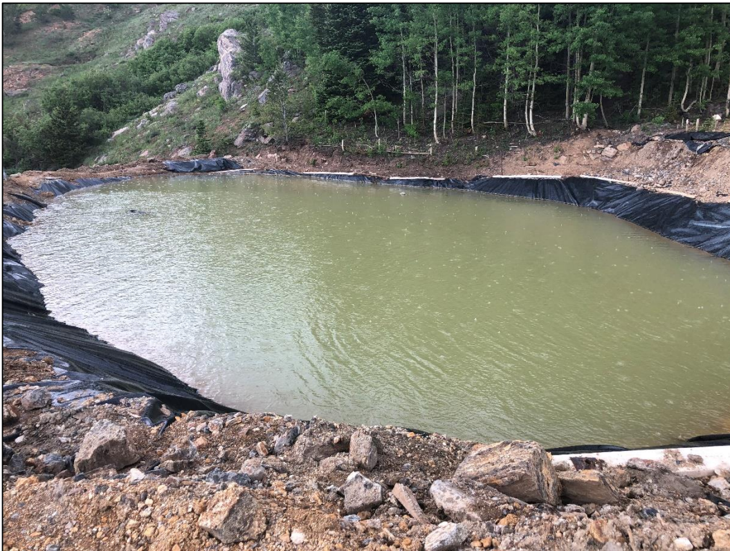
Photo 24. View looking southwest across Pond 3C (in Caribou Mine area) which was rehabilitated per TR-8. This is the largest and most downgradient of the three settling ponds.
