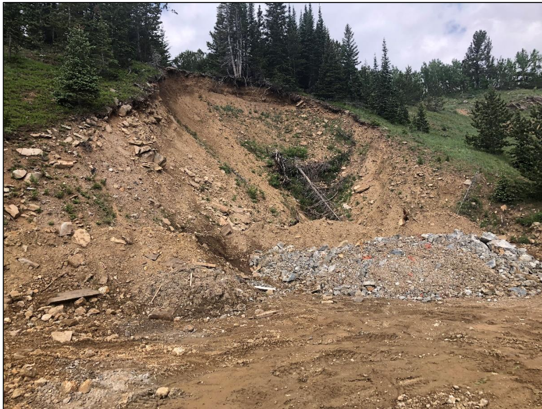
Photo 6. View looking west at New Cross Mine Decline Portal in Cross Mine area. Development of this portal was discontinued, leaving a partially excavated hillside with steep slopes.
