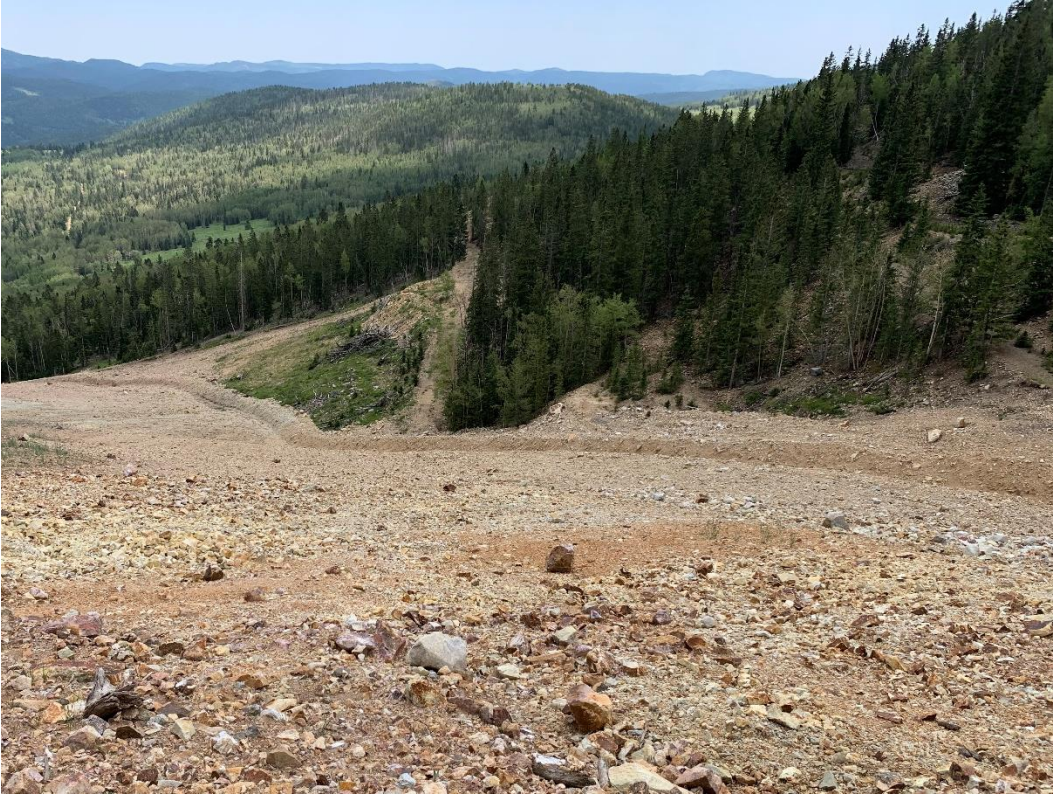
Photo 8 – Perimeter ditch on southern end of ECOSA
