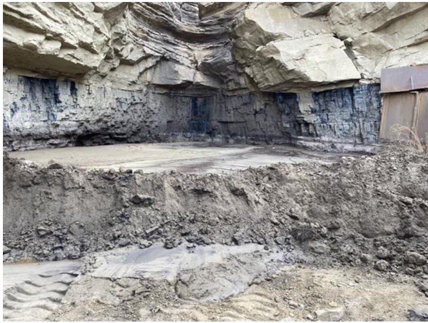
Photo 4: The eastern sump near the portals bench. The sump has filled and been overtopped by sediment from the areas upstream burned by a forest fire.
