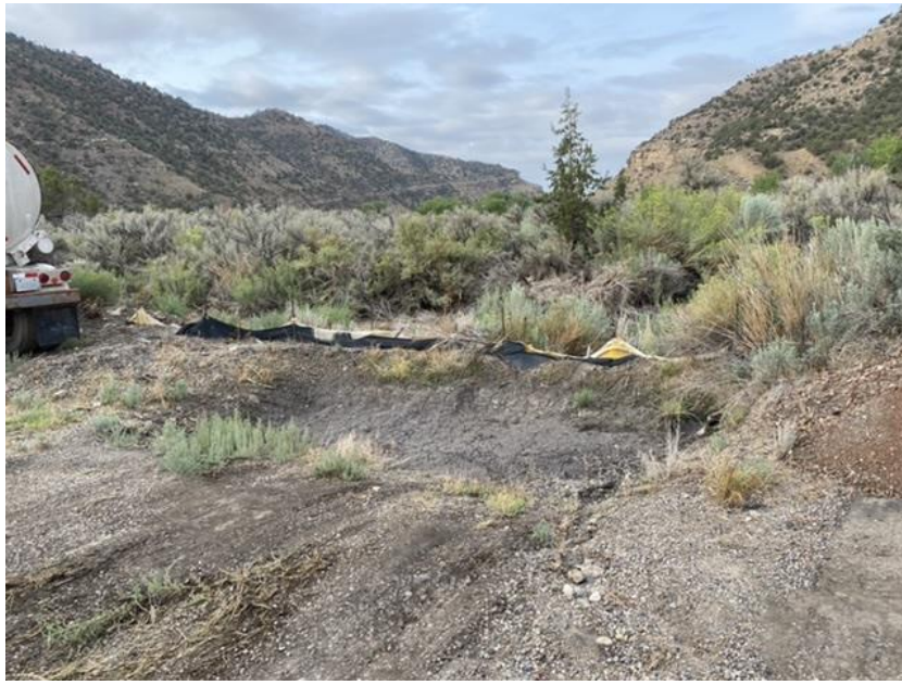
Photo 1: The sump south of the haul road near the mine office. The silt fence has fallen over and partly filled with sediment.
