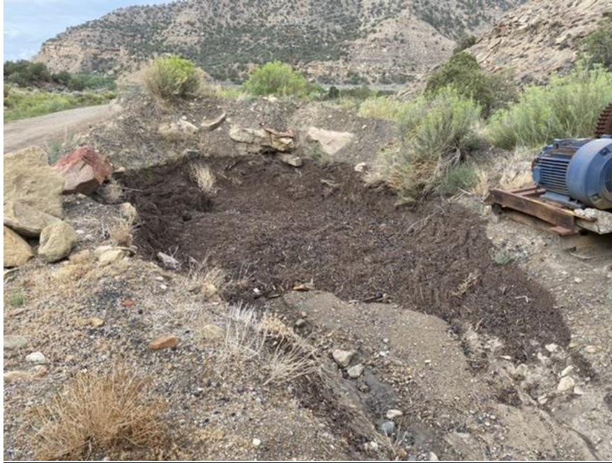
Photo 3: One of the sumps along the haul road upgradient of the sediment pond. The sump has filled with debris and sediment. The outlet to the sump was still clear.
