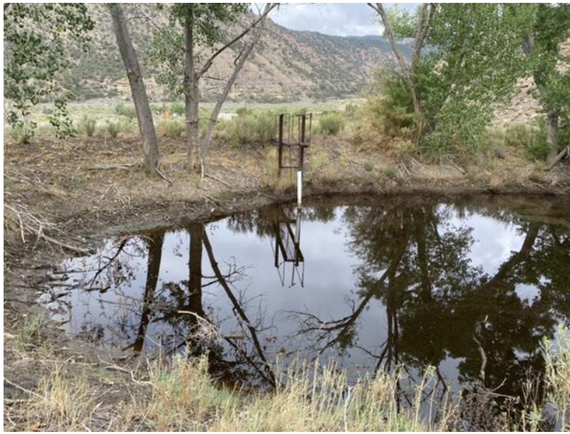
Photo 2: The sediment pond with impounded water. The water level was below the PVC riser for the outlet.
