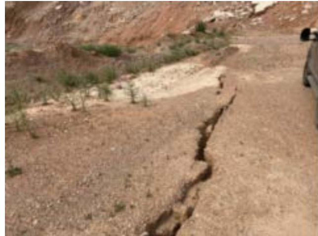
1. RECENT CRACKS ON PRODUCTION FLOOR AFTER RAIN
