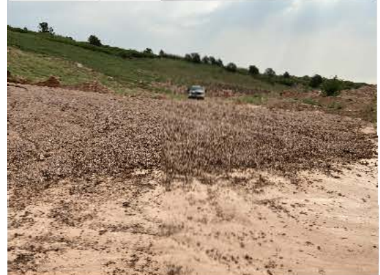
8. ERODED MATERIAL BELOW CULVERT
