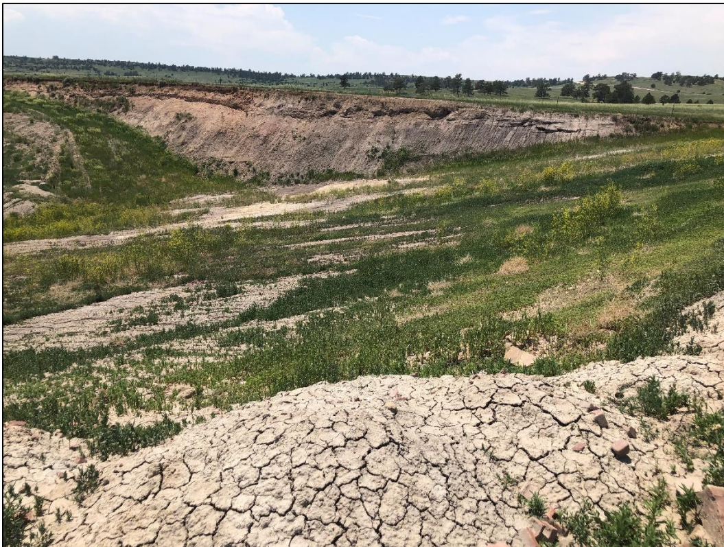
Photo 10. View looking southwest across northern edge of larger excavation in southern half of Phase III permit area. Note unbackfilled portion of western highwall visible in background.
