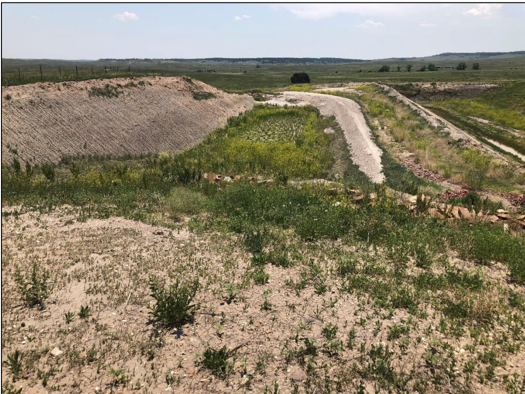
Photo 12. View looking south across smaller excavation in southern half of Phase III permit area. Note eastern highwall (at left) which is approximately 20 feet in height with 1H:1V slopes.
