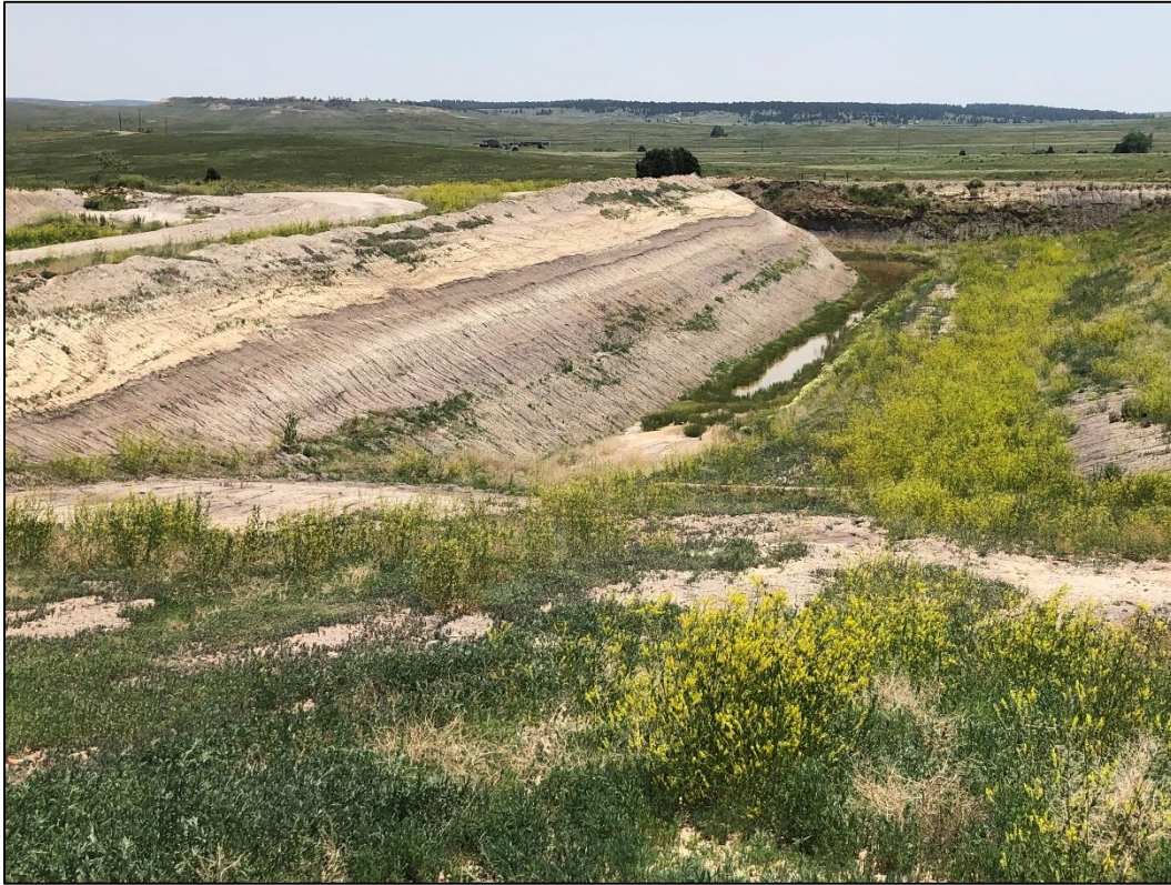
Photo 9. View looking south at eastern highwall of larger excavation in southern half of Phase III permit area, which is approximately 25 feet in height with 2H:1V slopes.
