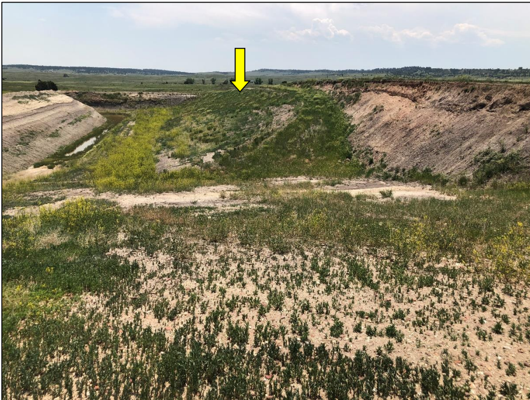
Photo 8. View looking south across larger excavation in southern half of Phase III permit area. Note backfilled portion of western highwall (indicated) with 3H:1V or flatter slopes. Also note portion of western highwall that remains with 1H:1V slopes (at right).
