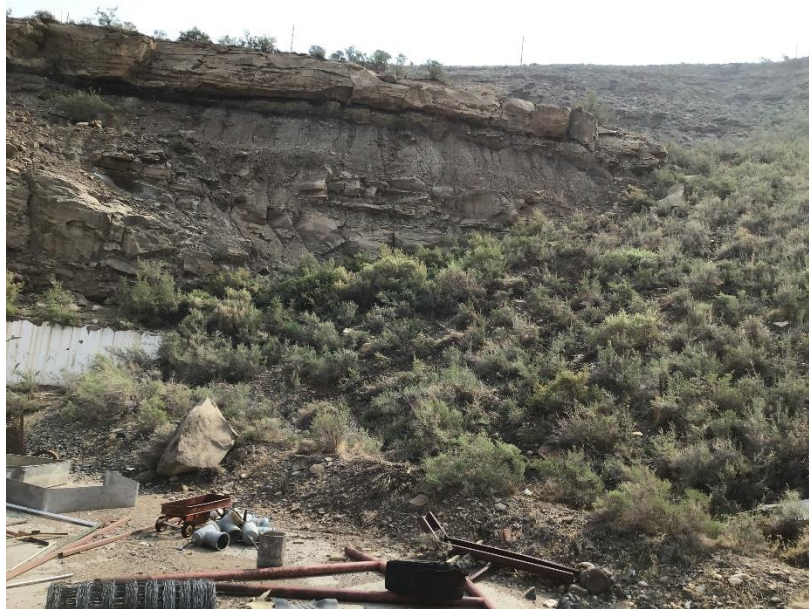
Photo 1: The reclaimed mine portals. No water was observed seeping from the reclaimed slope or flowing out of the French drain.
