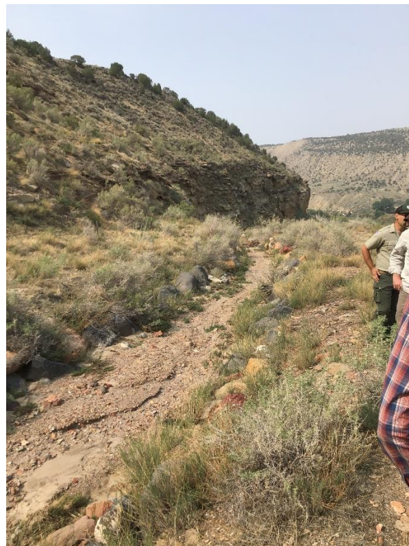
Photo 2: The upland diversion ditch for the reclaimed refuse pile.
