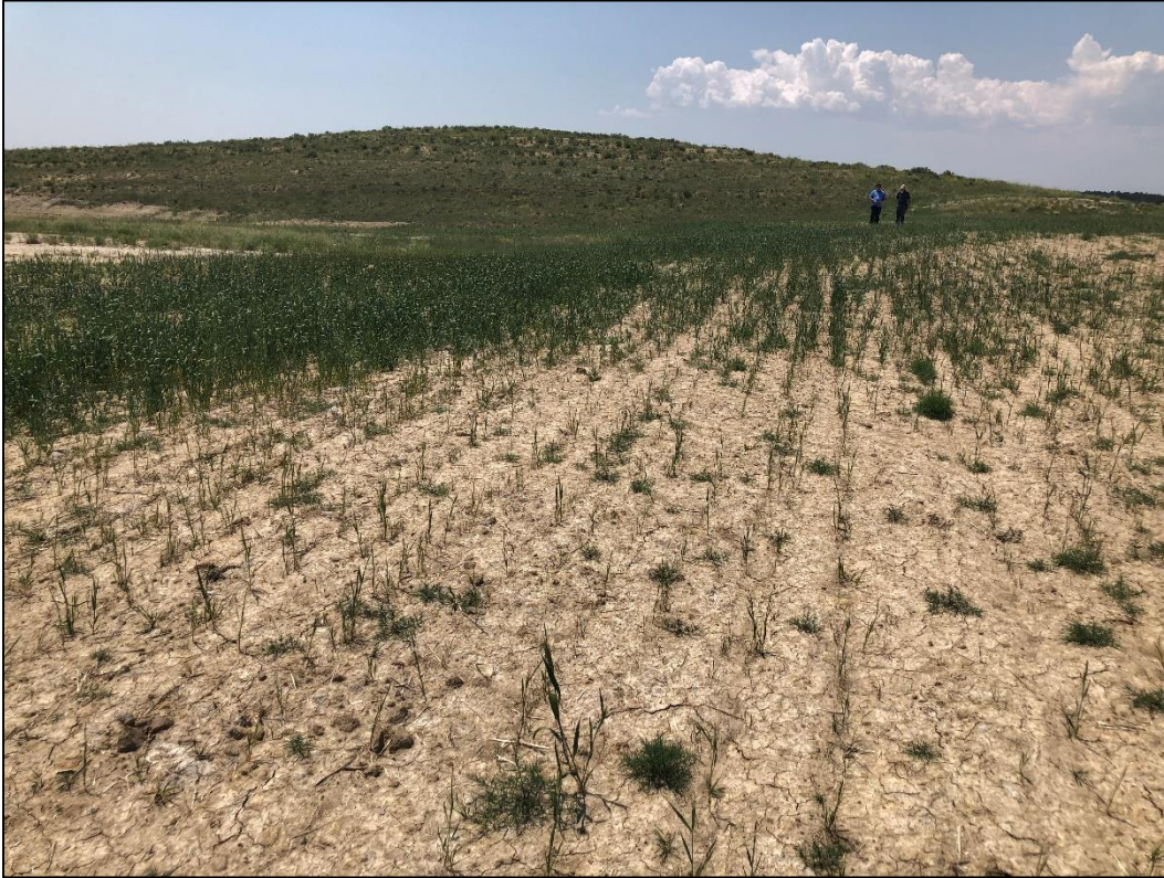
Photo 11. View looking south across phase 2 and 3 pit area (in northern portion of permit area), showing slopes graded to 3H:1V or flatter. Note area in foreground with very sparse vegetative cover which may require additional seeding.
