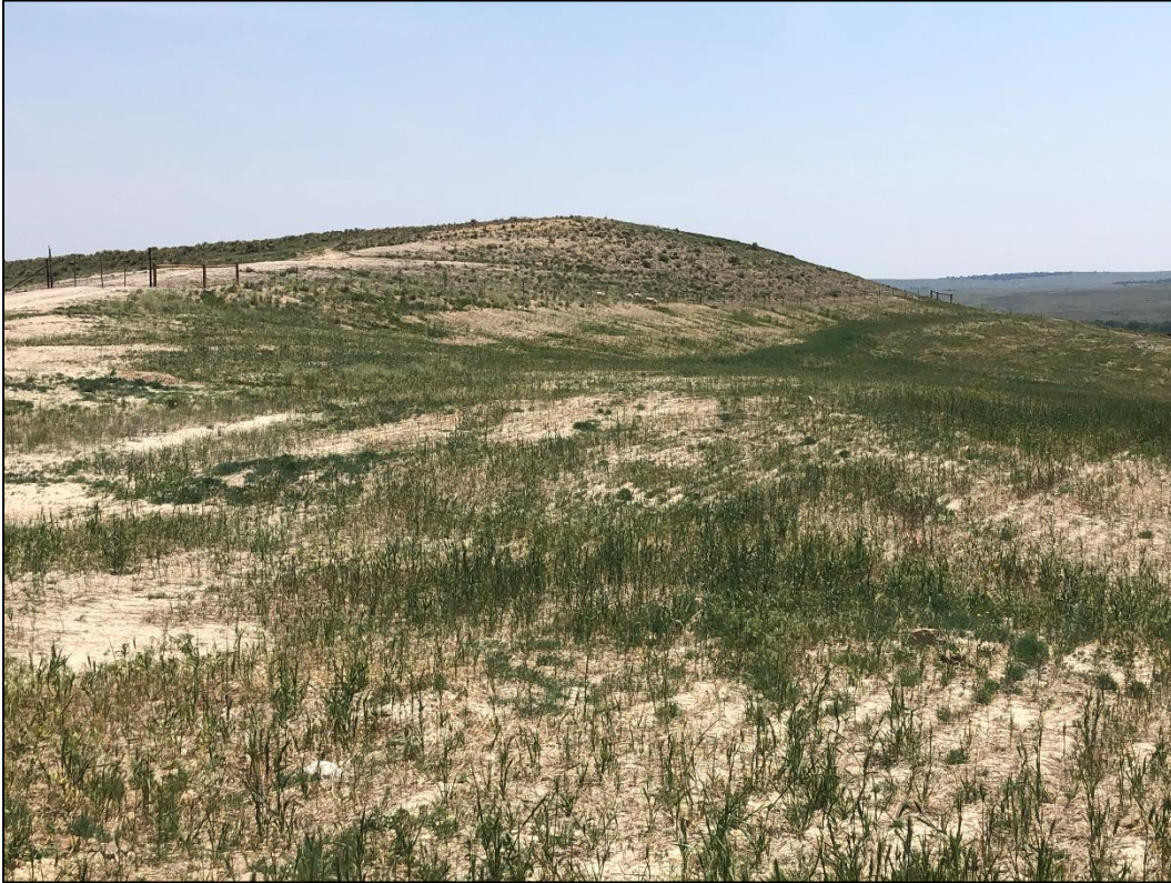
Photo 9. View looking northeast across phase 2 and 3 pit area (in northern portion of permit area), showing slopes graded to 3H:1V or flatter. Note sparse vegetative cover in some areas which may require additional seeding.
