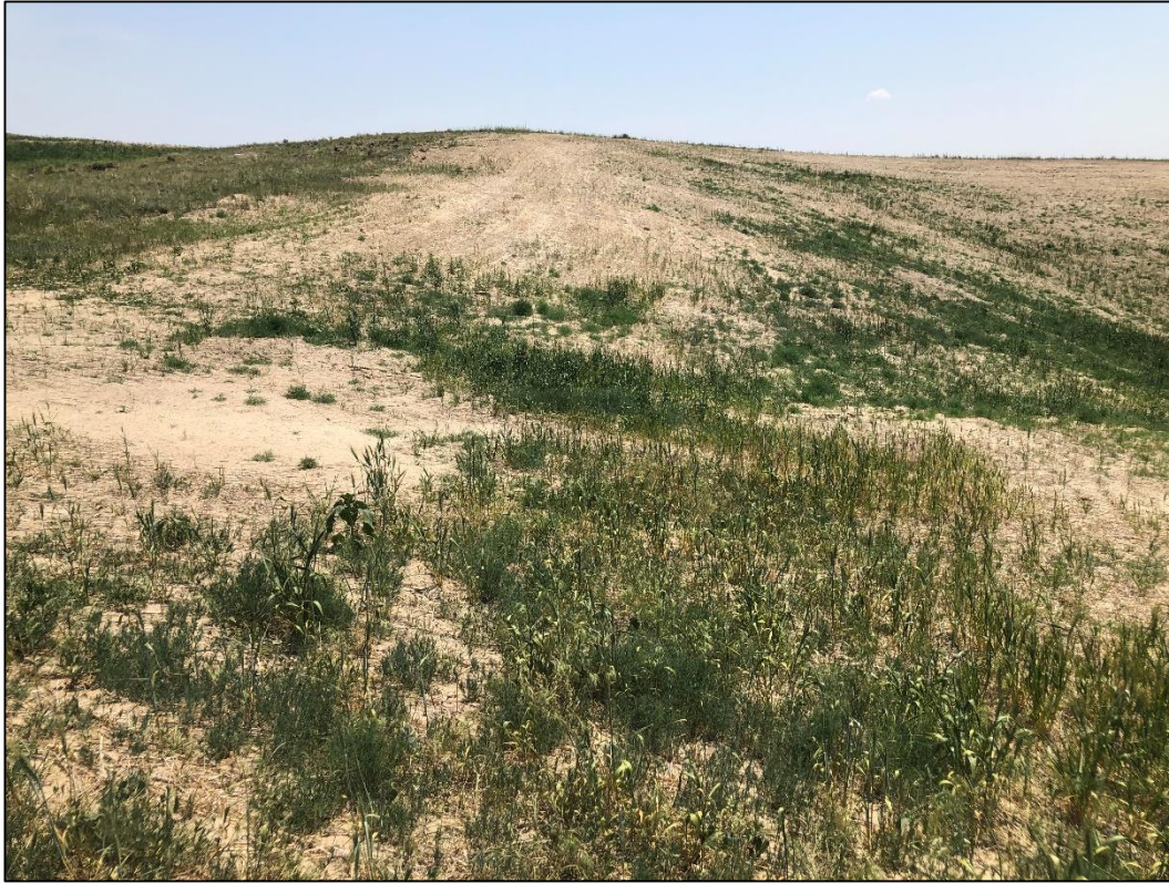
Photo 3. View looking southeast across northern slope of phase 4 pit (in southern portion of permit area), showing slopes graded 3H:1V or flatter. Note sparse vegetative cover along top of slope which may require additional seeding.
