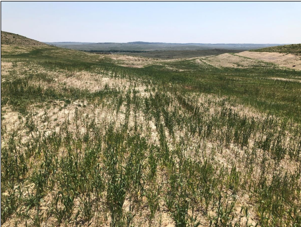
Photo 8. View looking east across phase 2 and 3 pit area (in northern portion of permit area), showing slopes graded to 3H:1V or flatter. Note sparse vegetative cover in some areas which may require additional seeding.
