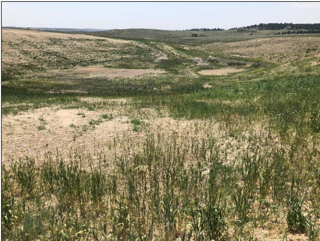
Photo 4. View looking southeast across phase 4 pit (in southern portion of permit area), showing slopes graded to 3H:1V or flatter. Note sparse vegetative cover along top of slopes and in a few areas on the pit floor which may require additional seeding.
