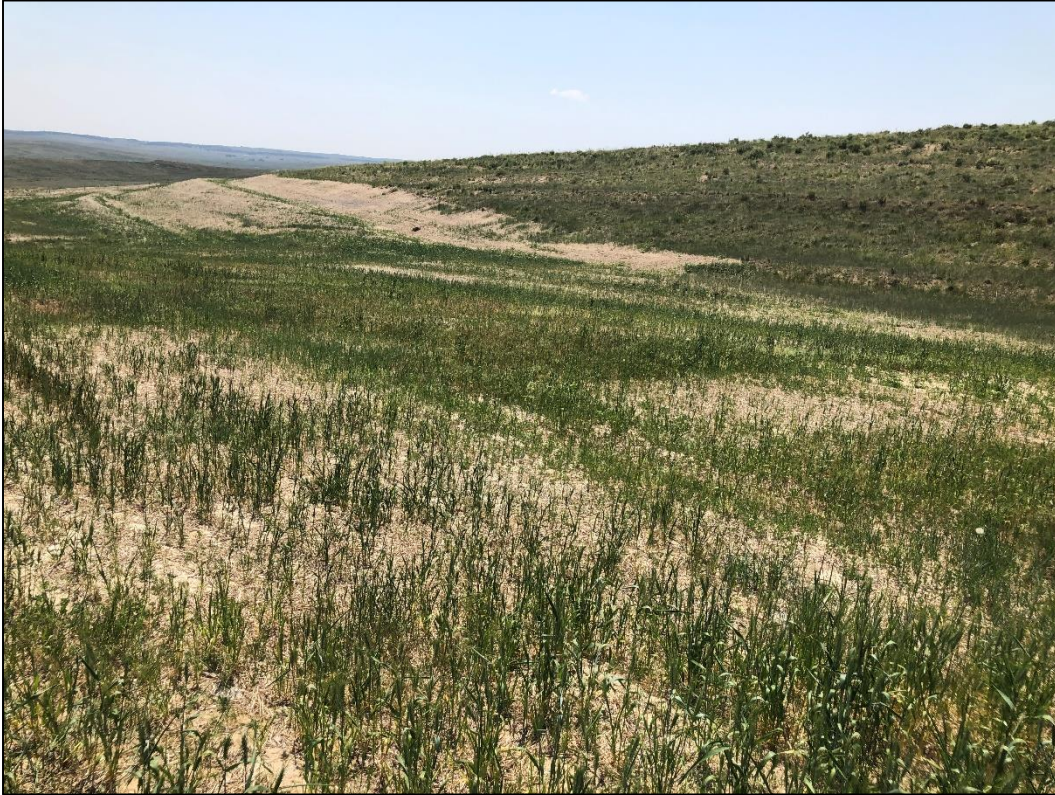
Photo 7. View looking southeast across phase 2 and 3 pit area (in northern portion of permit area), showing slopes graded to 3H:1V or flatter. Note sparse vegetative cover in some areas which may require additional seeding.
